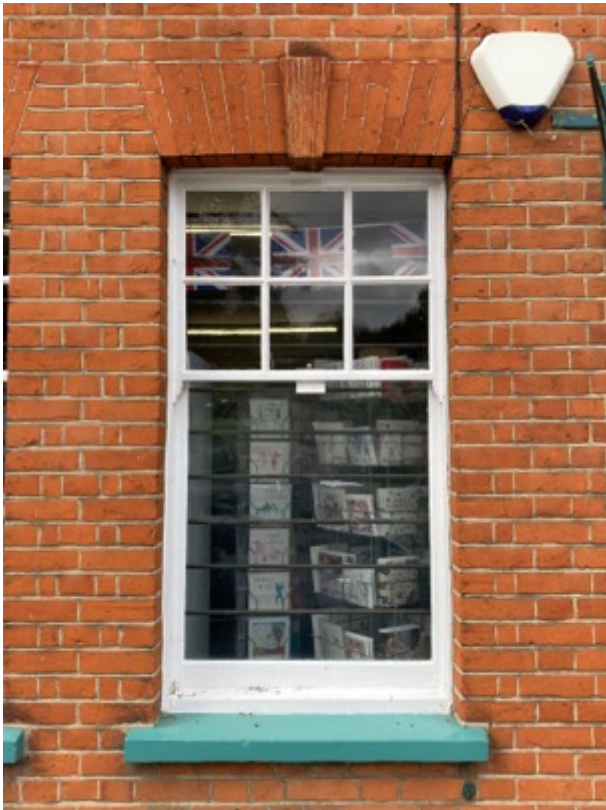
Existing Sash Window
