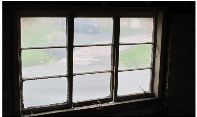
The windows are single glazed wooden framed, and none are intact
