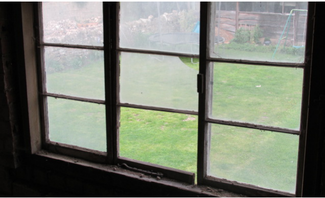
The windows are single glazed wooden framed, and none are intact
