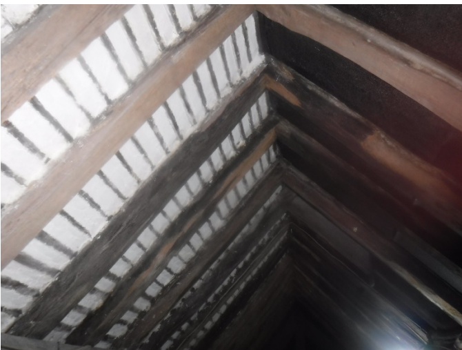
Photo 5. Loft void – torching and felt lined
