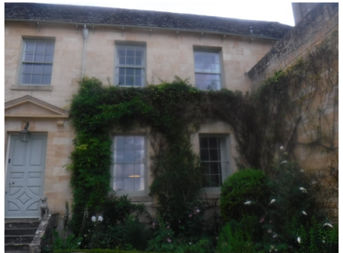
Photo 4. Window repairs / replacements beyond parapet wall on right hand side
