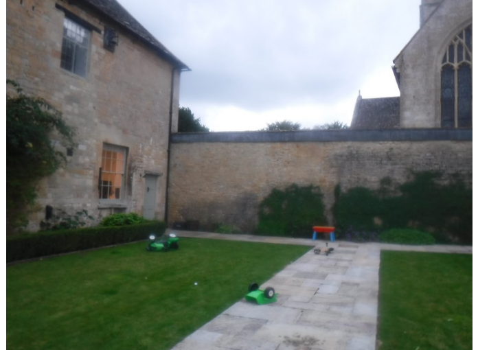
Photo 2. Section of lead flashing to be subject to works
