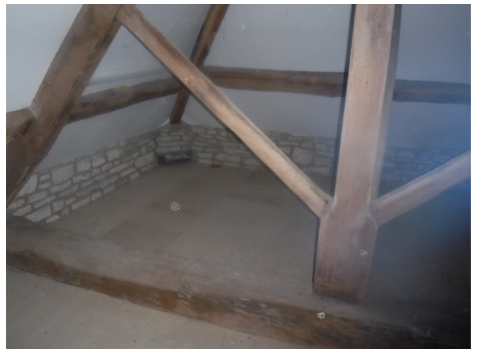
Photo 6. Loft void – separate enclosed section
