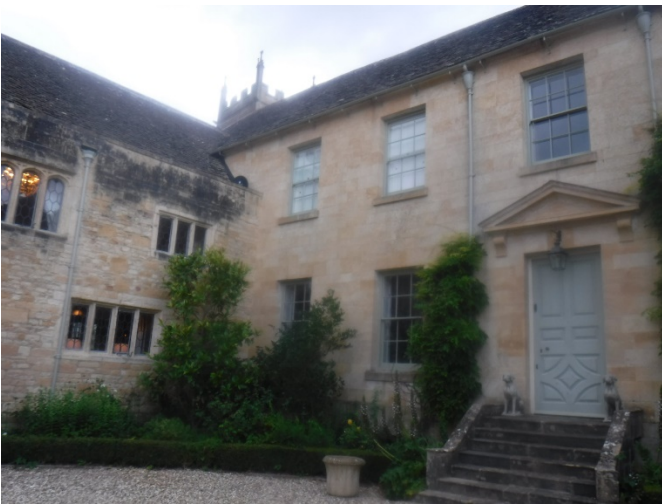
Photo 3. Rainwater goods on left hand side to be subject to works
