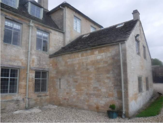
Photo 1. Eastern extension to be subject to works
