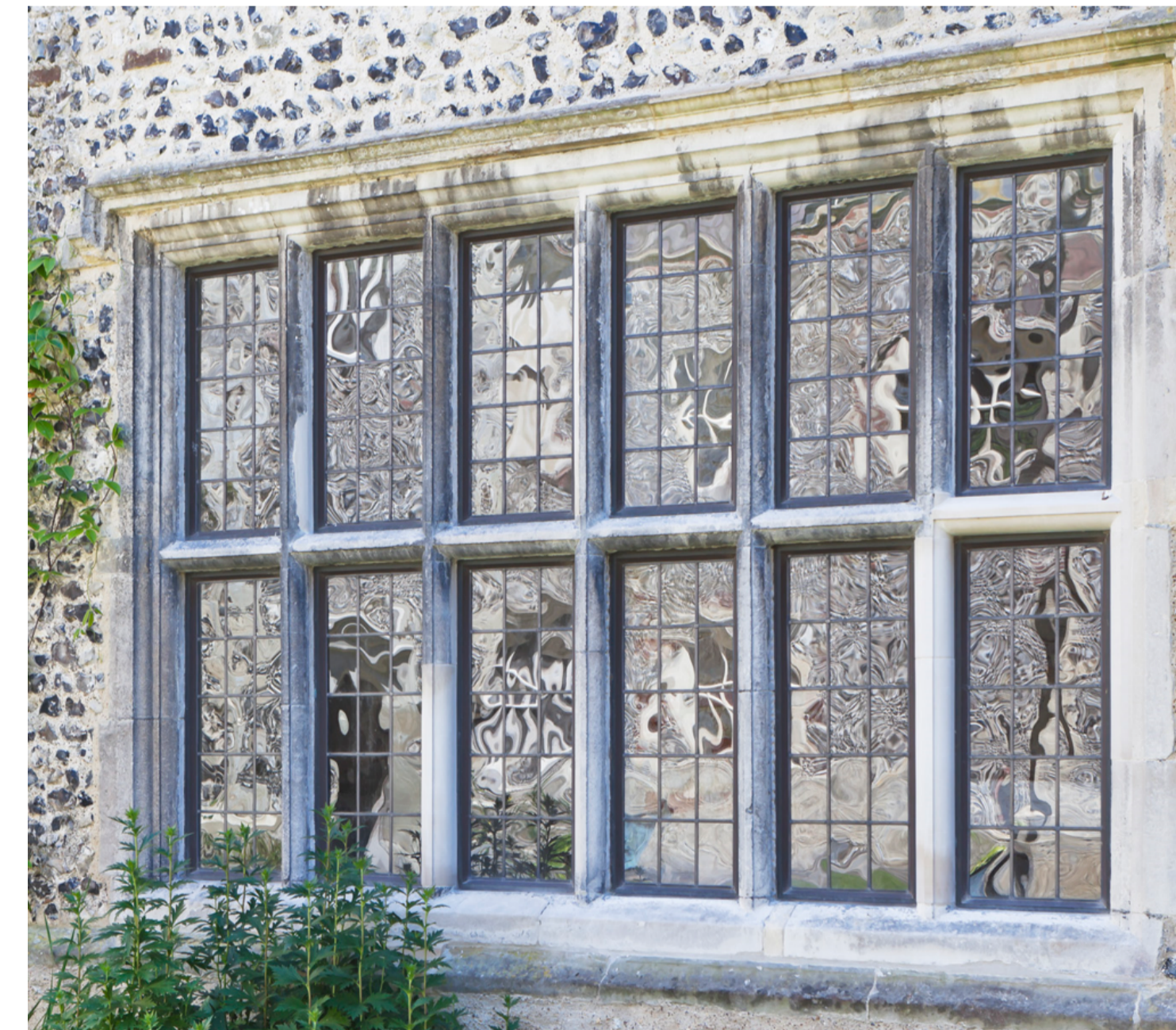
PROPOSED BRONZE CASEMENT WINDOW (HERITAGE PROFILE) WITH KILN DISTORTED GLASS
