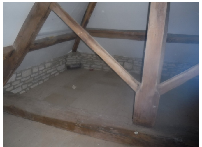
Photo 6. Loft void – separate enclosed section
