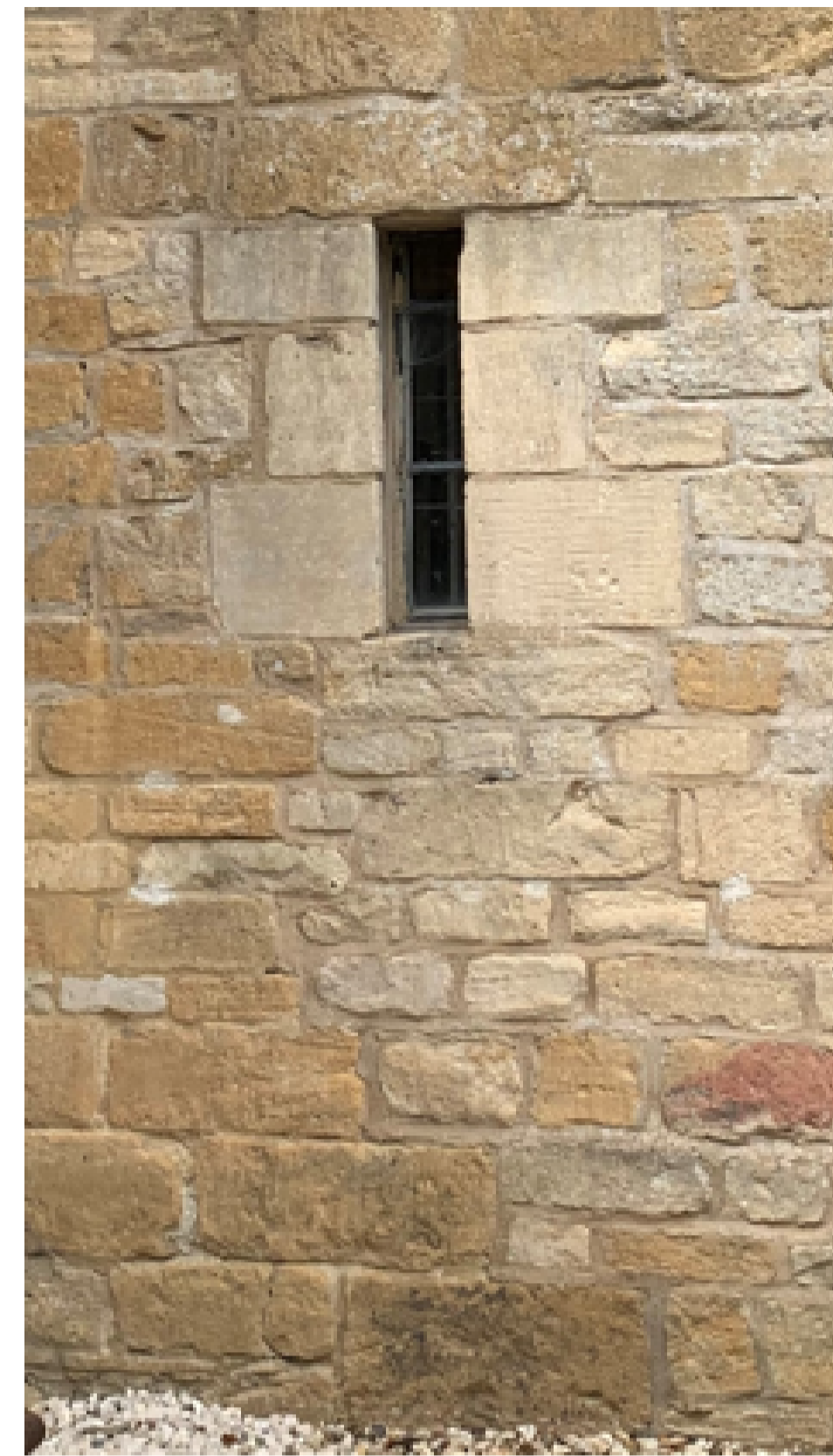
PHOTO OF EXISTING EXTERNAL ELEVATION
