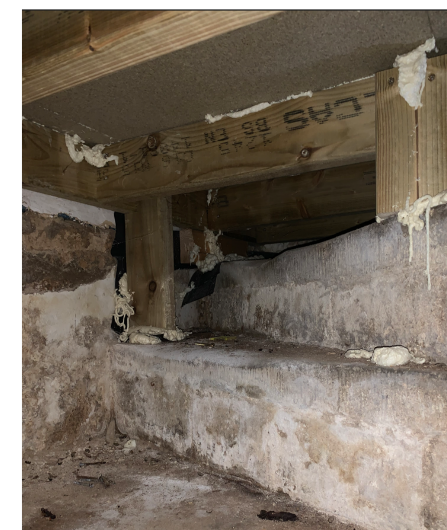
PHOTO 3 - EXISTING FLOOR STRUCTURE IN BASEMENT
