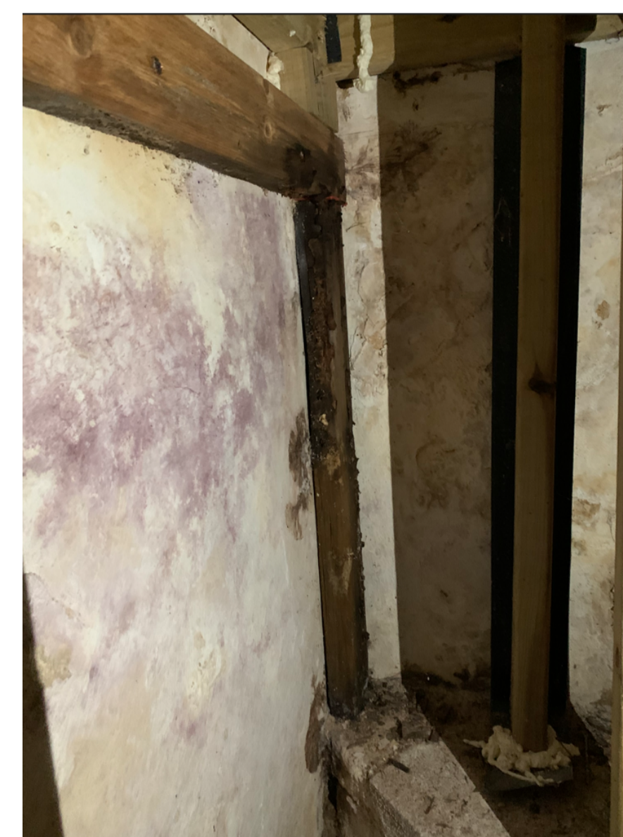
PHOTO 2 - EXISTING FLOOR STRUCTURE IN BASEMENT
