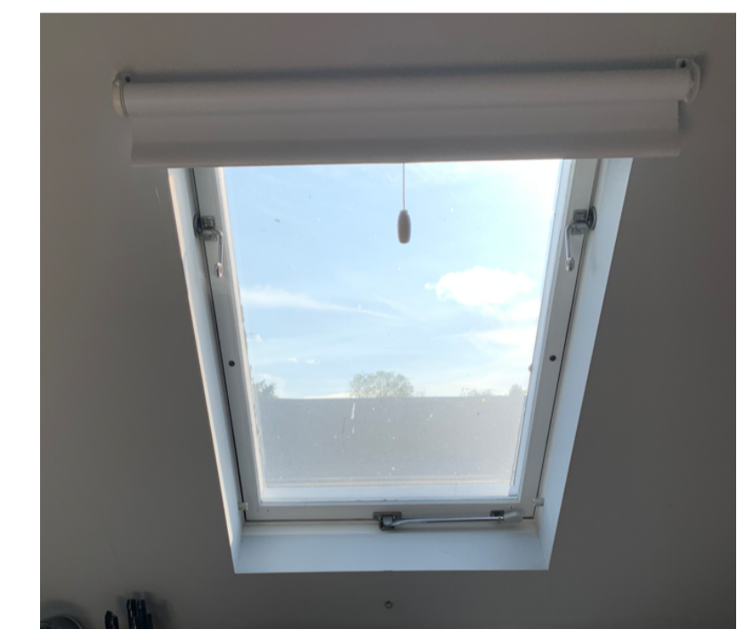
INTERNAL CONDITION OF EXISTING ROOFLIGHT
