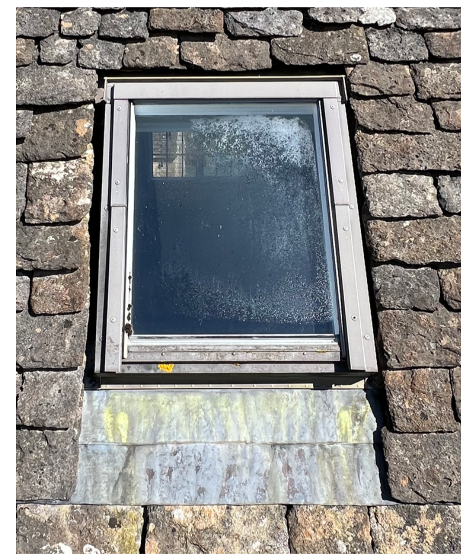
EXTERNAL CONDITION OF EXISTING ROOFLIGHT
