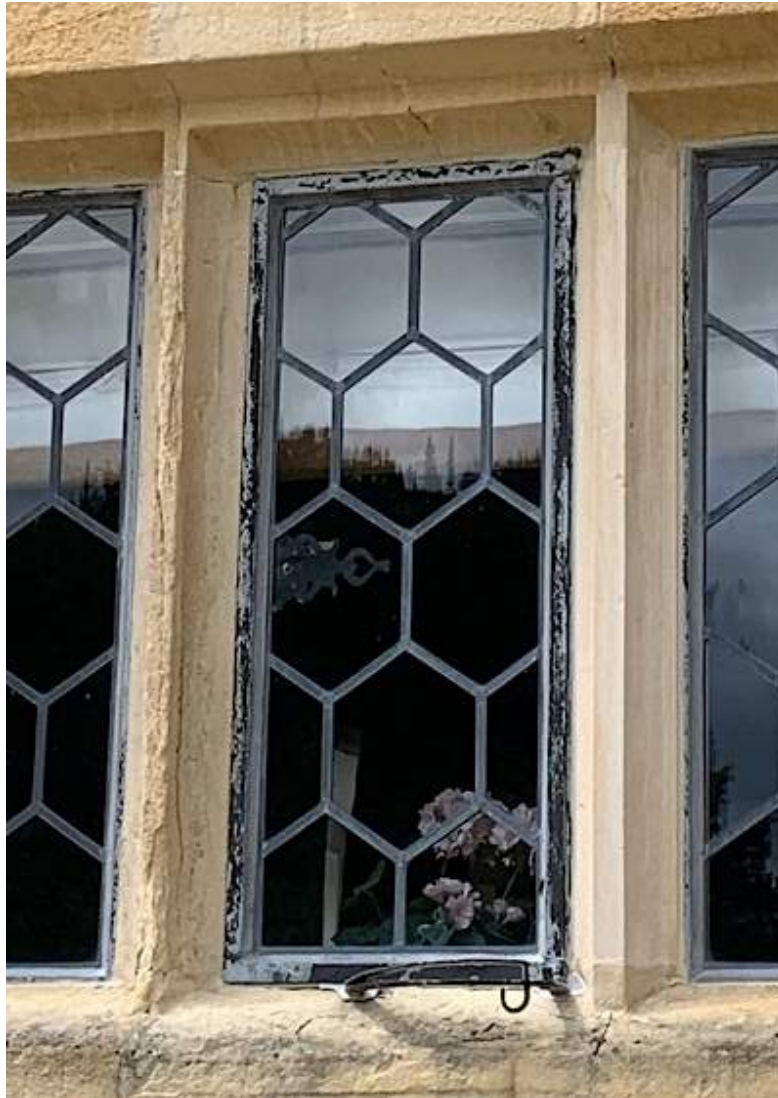
Figure 15 Eastern mullioned window.
