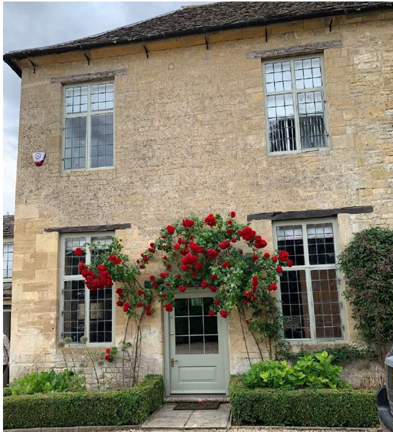
Figure 3 Eastern end of north front, with historic casements at ground floor, & modern replicas at first floor.
