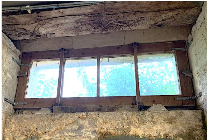
Figure 19 Detail of basement window from the interior.
