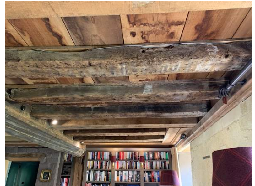
Figure 23 South-west wing, ground floor ('snug') ceiling.
