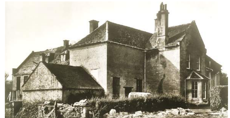
Figure 2 Mid-20 th century view from the north-east.
