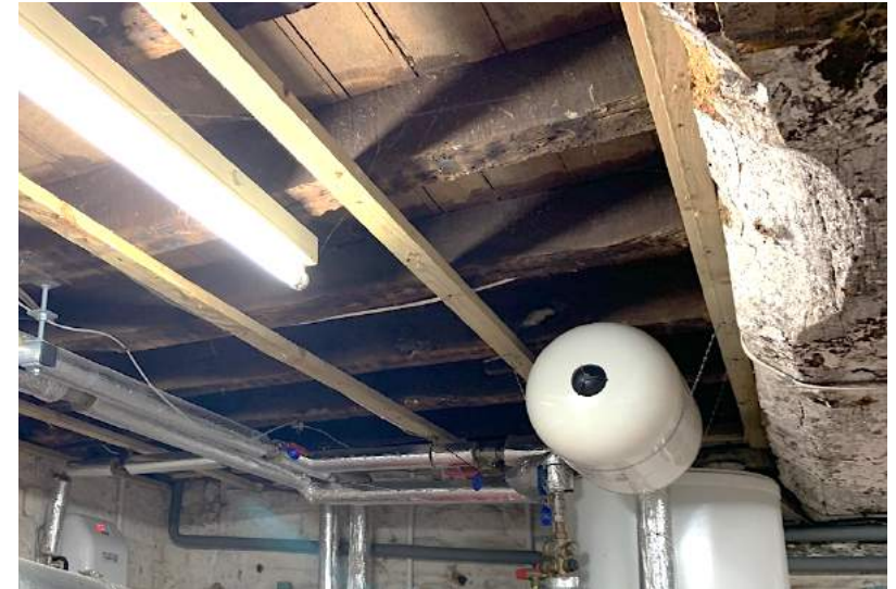
Figure 22 Ceiling of basement beneath dining room.
