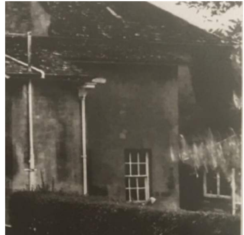
Figure 27 Mid-20th century photograph, with lead-to just visible to right.
