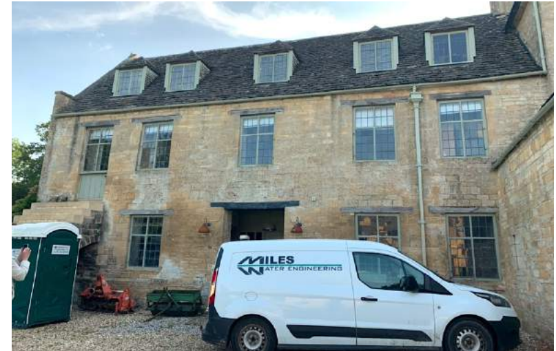
Figure 1 Historic casements on the east front of south-east wing (dormers are replicas, with uncharacteristically wide cheeks).
