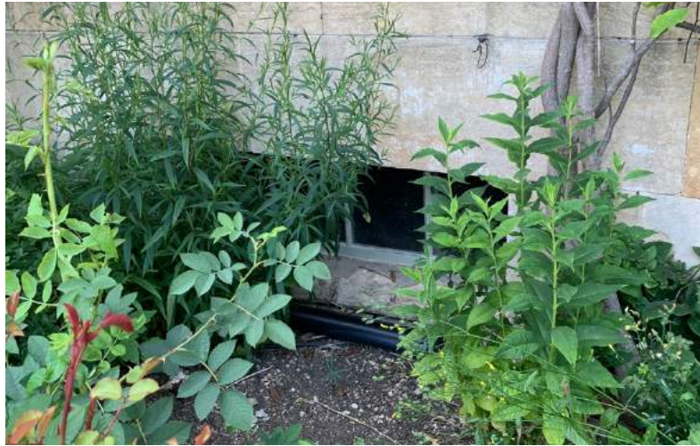
Figure 18 Detail of basement window from the exterior.
