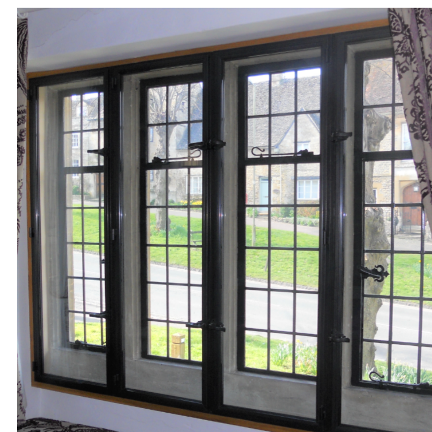
PROPOSED SECONDARY DOUBLE GLAZING
