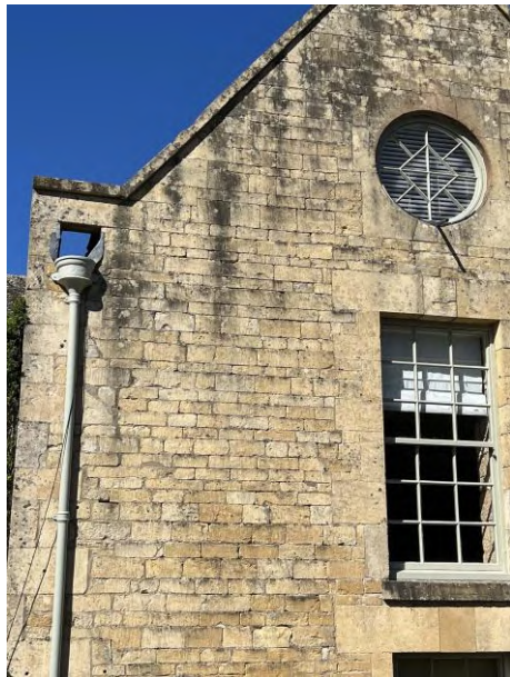
Above: View of east wing gable. The overhang on the gable copings is visible. There is black staining to the stone façade where pointing has come away between the copings.
