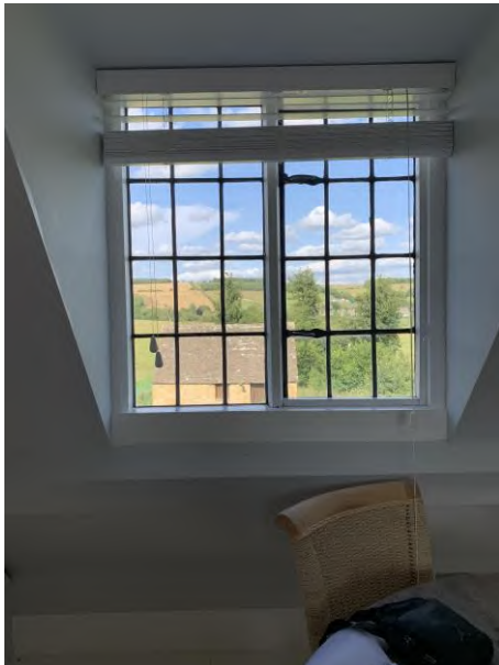
Above left: Typical dormer window to the Studio, comprising single-glazed leaded lights.
