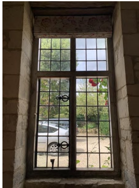
Figure: Existing historic cruciform window in the Well Room, with single-glazed leaded lights.
