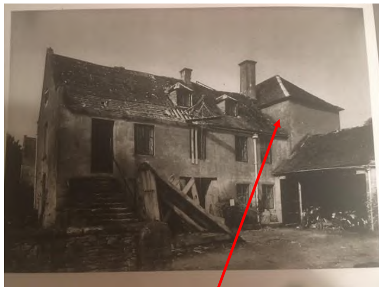
East Wing: East Elevation circa 1970. No windows are visible at first floor level to the area now designed as Laundry Room. Note that only two dormers at Attic level were existing (area identified
