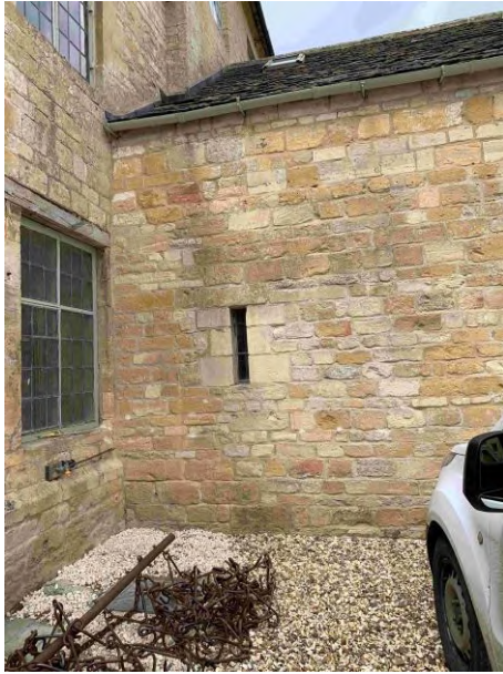
Above Left: Cottage Bathroom window WG13 as existing – exterior view
