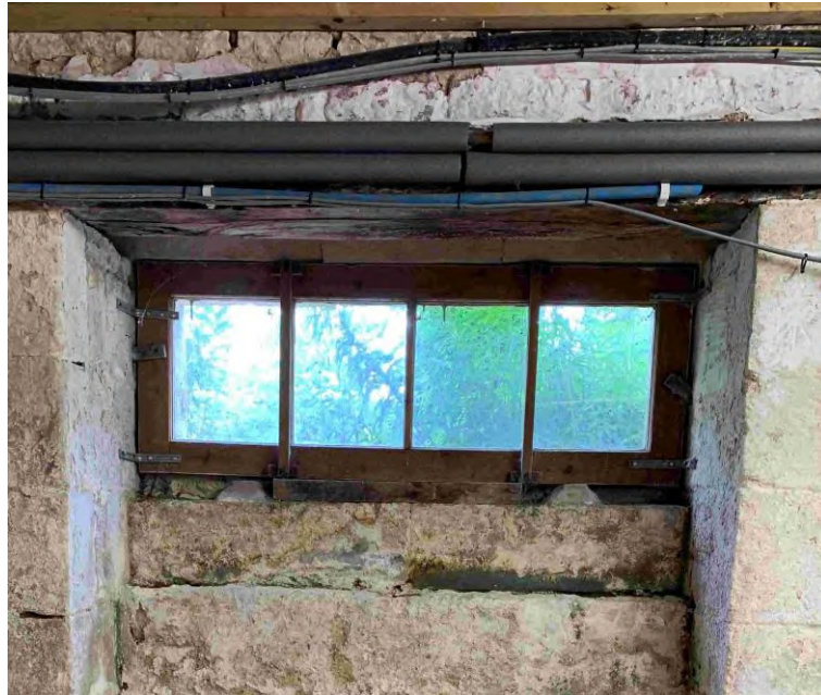
Above: Existing Basement Window
