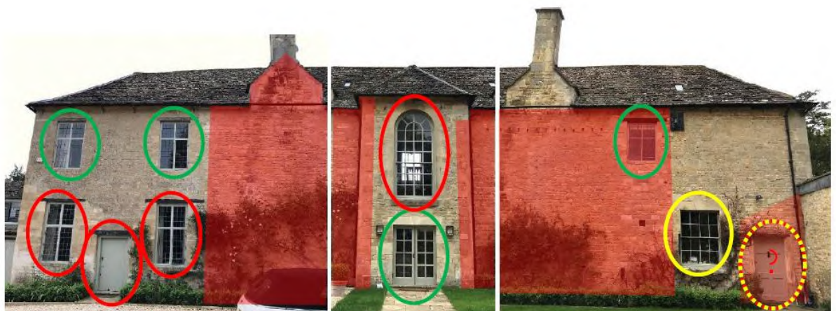
Figure 1 North front, extent of elevation covered by other structures until the latter half of the 20 th century. Encircled openings: 18 th century; 19 th century; 20 th century (n.b. first-floor right appears to contain an 18 th -century casement reused from elsewhere in the building).
