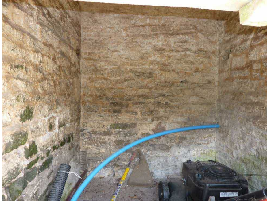
Photograph 9 Interior space as viewed from open frontage in East Elevation.
