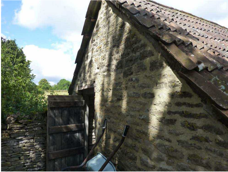
Photograph 3 View on to gable end wall of South Elevation.
