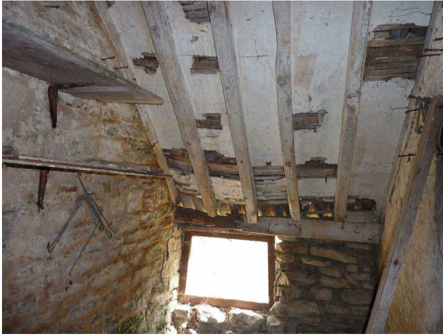
Photograph 5 View to underside of roof structure within building interior (south side).
