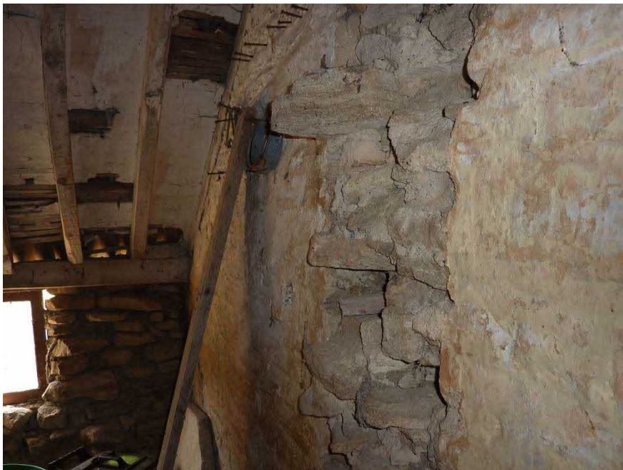
Photograph 6 Evidence of wall removal within building interior adjacent to South gable.
