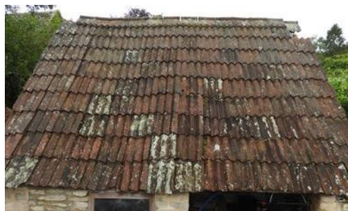
Figs. 4 Ridge and roof tiles to the east
