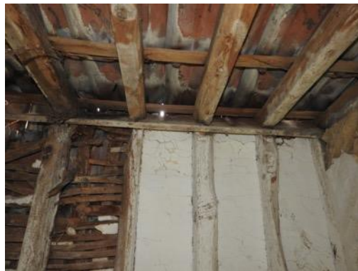
Fig. 7 Partially lined room against the south gable wall
