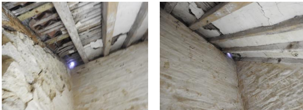
Figs. 10 & 11 West room against the north gable wall
