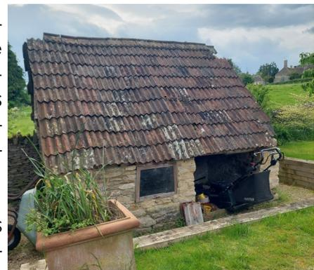
nally divided into four small spaces. It was built off the stone field wall on the west boundary of the plot, with a very low eaves facing into the garden. The east elevation is partly open to the interior, and it is evident from the pattern of the stonework that originally the whole of the east elevation would have been open.
