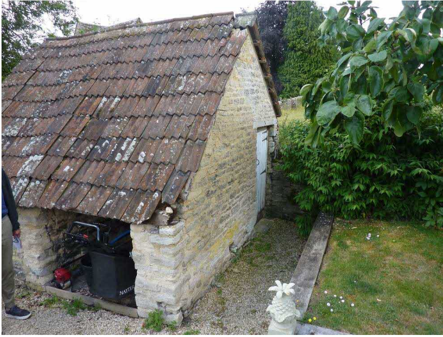
Photograph 1 View on to gable end wall of North Elevation
