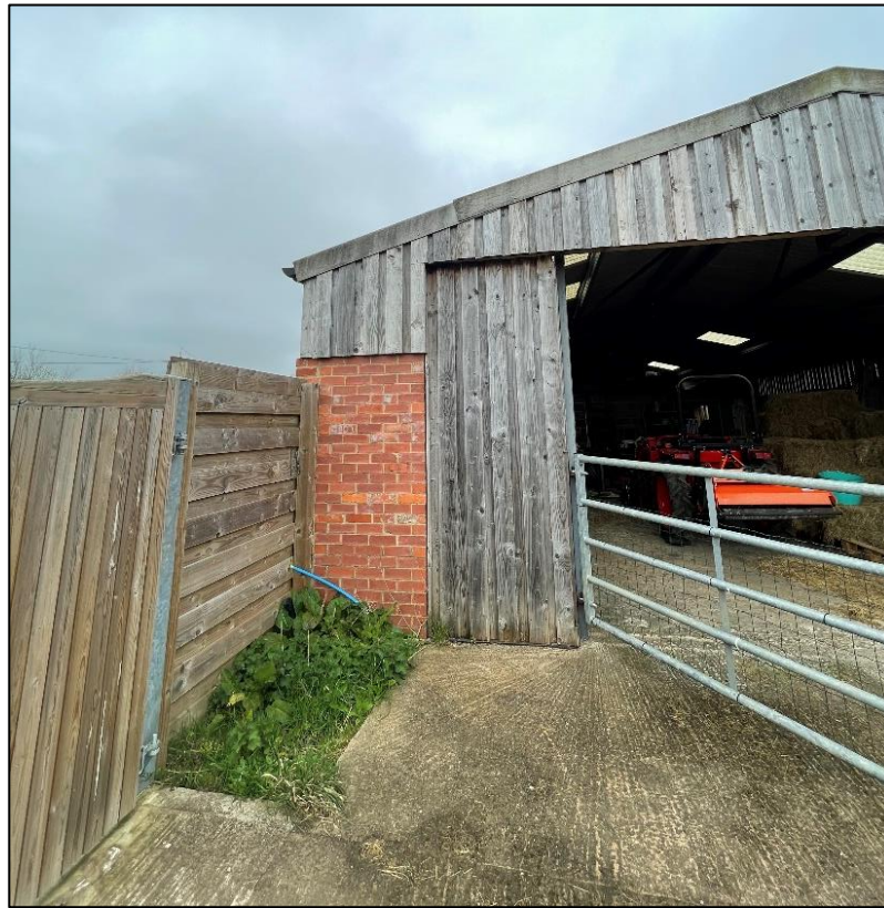
Figure 2: Western elevation of the barn at Westbrook Barns
