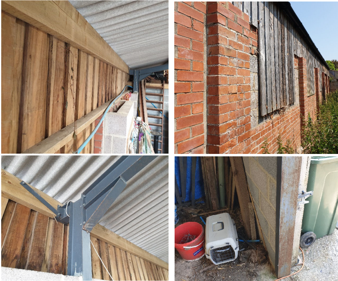
Figure 5 Perimeter wall construction
