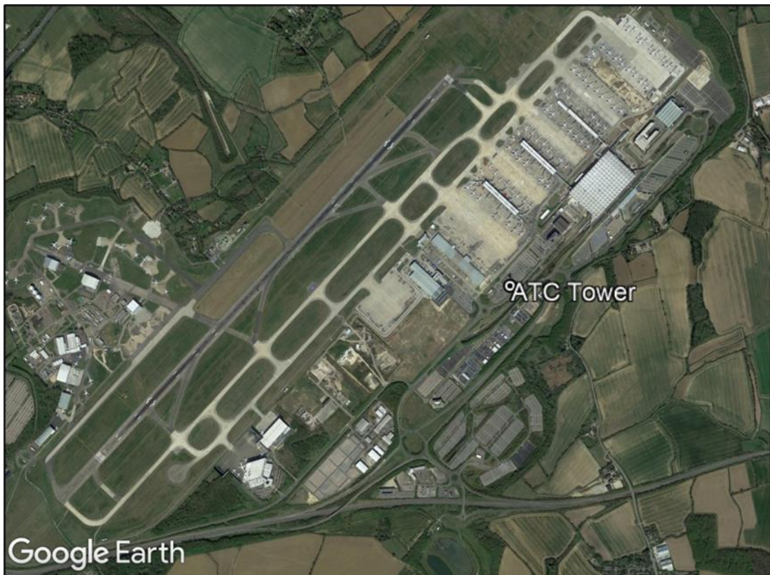
Figure 10 Location of the ATC Tower within London Stansted Airport
