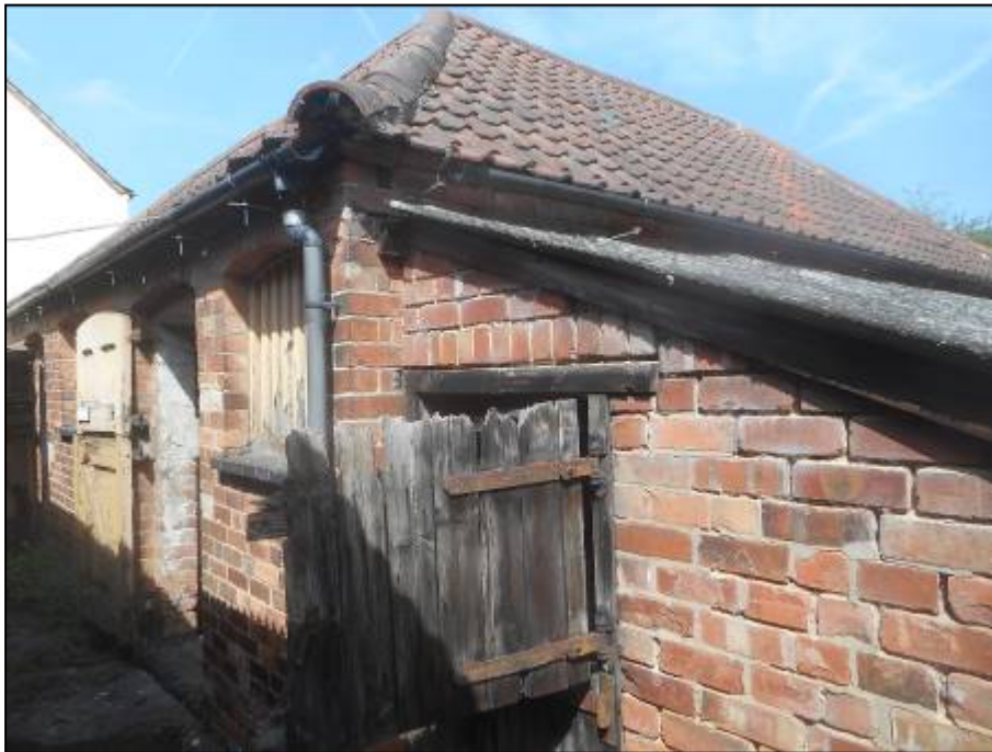
Photograph 2 - Southern aspect of Building 1
