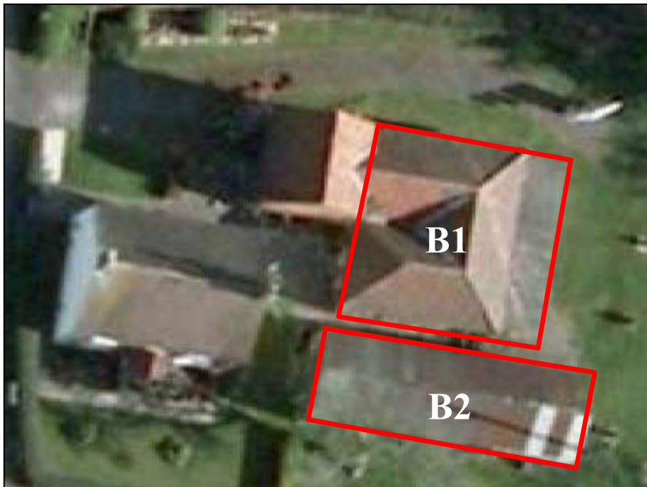
Plate 1 - Aerial view of building with sections surveyed in red
