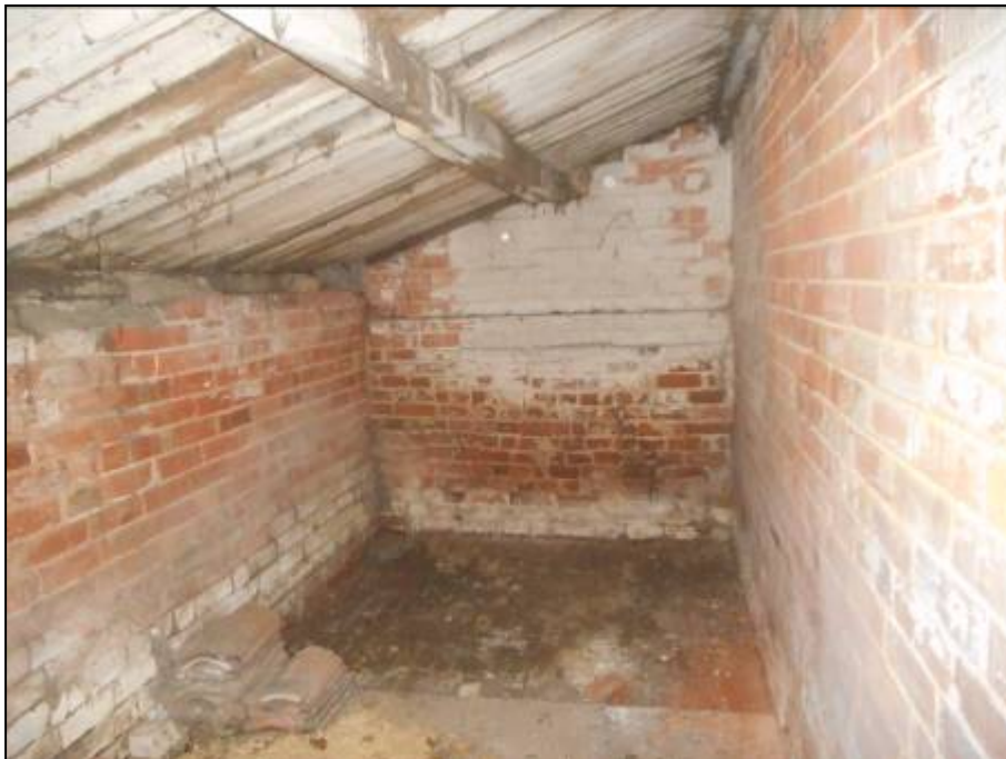
Photograph 3 - North-eastern internal section of Building 1
