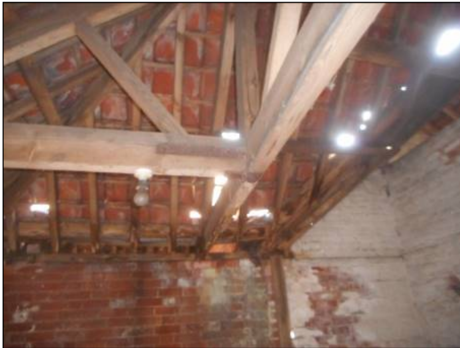
Photograph 8 - South-western internal section of Building 1
