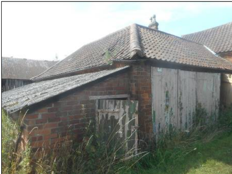
Photograph 1 - Northern aspect of Building 1
