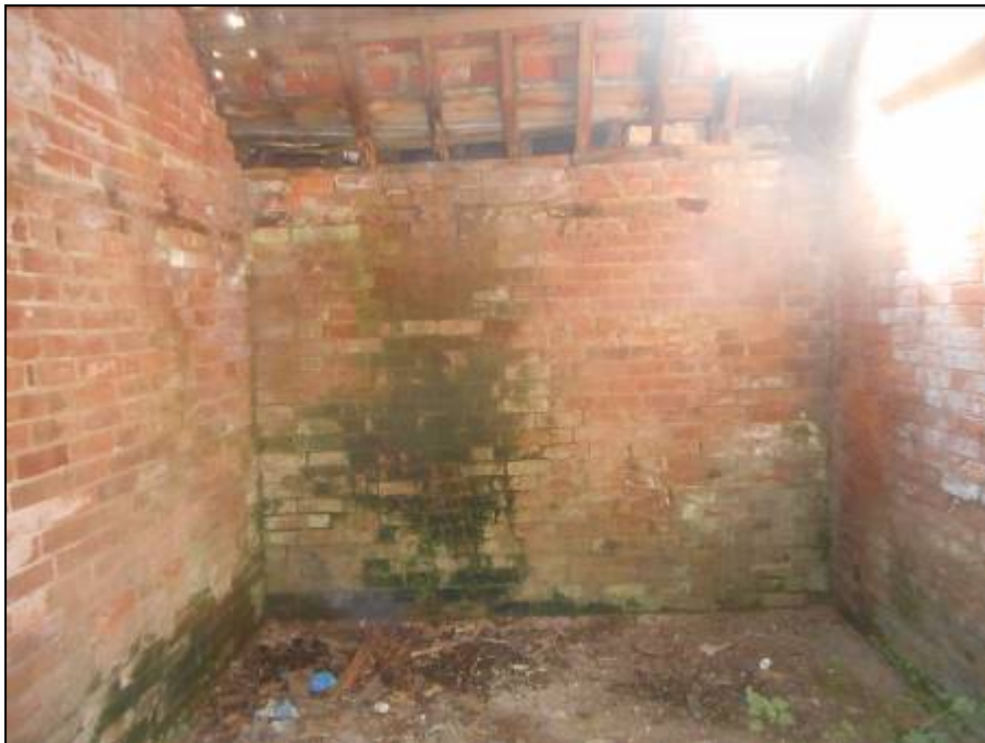
Photograph 5 - North-western internal section of Building 2
