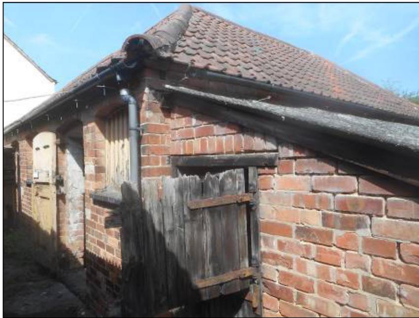
Photograph 2 - Southern aspect of Building 1
