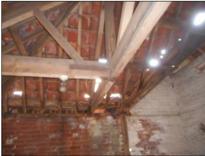
Photograph 8 - South-western internal section of Building 1
