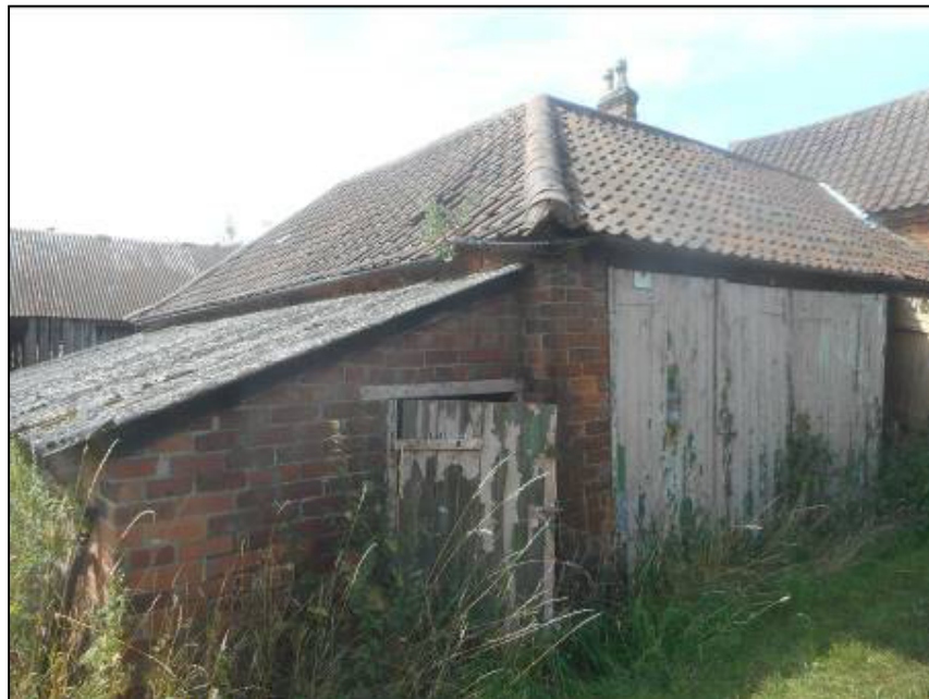
Photograph 1 - Northern aspect of Building 1
