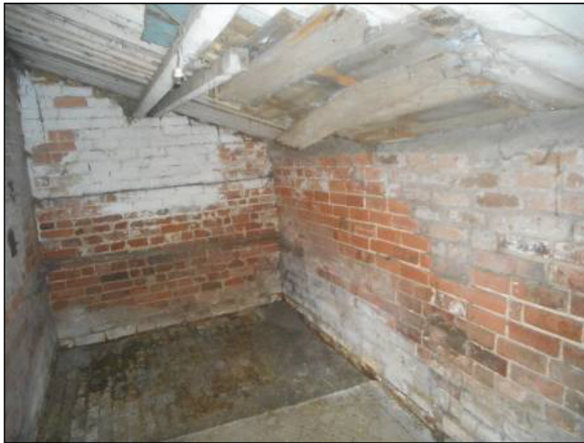
Photograph 6 - South-eastern internal section of Building 1
