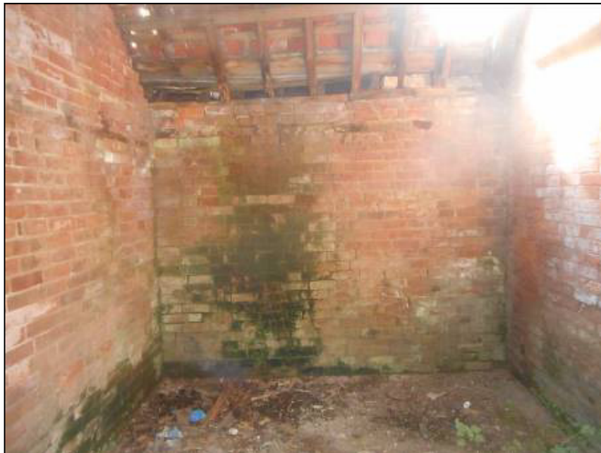
Photograph 5 - North-western internal section of Building 2
