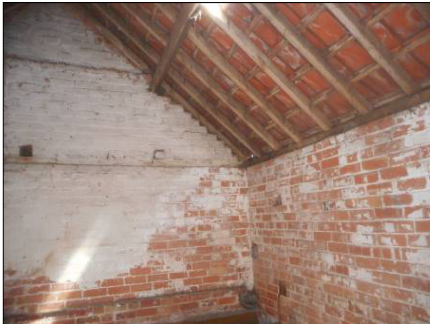
Photograph 7 - Central internal section on southern side of Building 1
