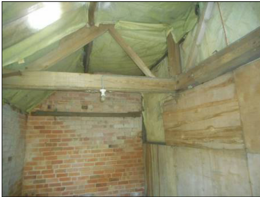
Photograph 4 - Central internal section on northern side of Building 1
