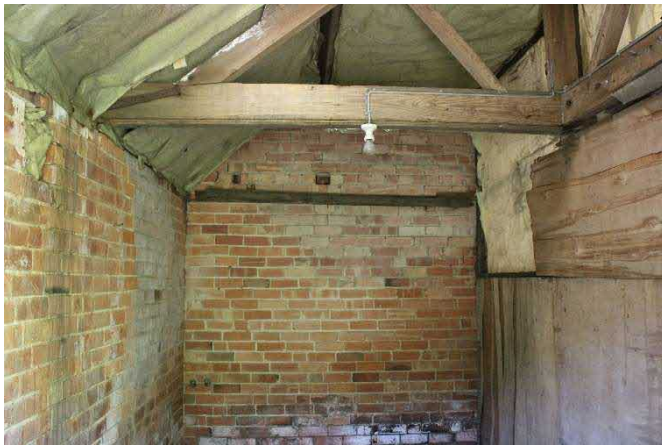
Figure 15. General view of rearmost bay
