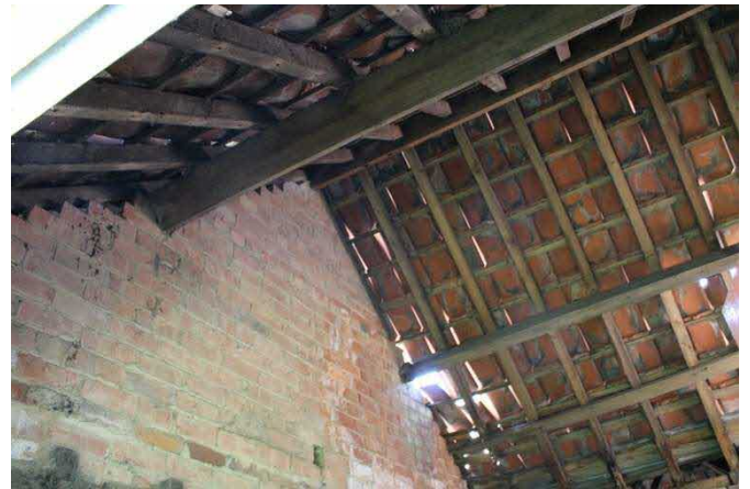
Figure 16. Roof structure to single storey barr
