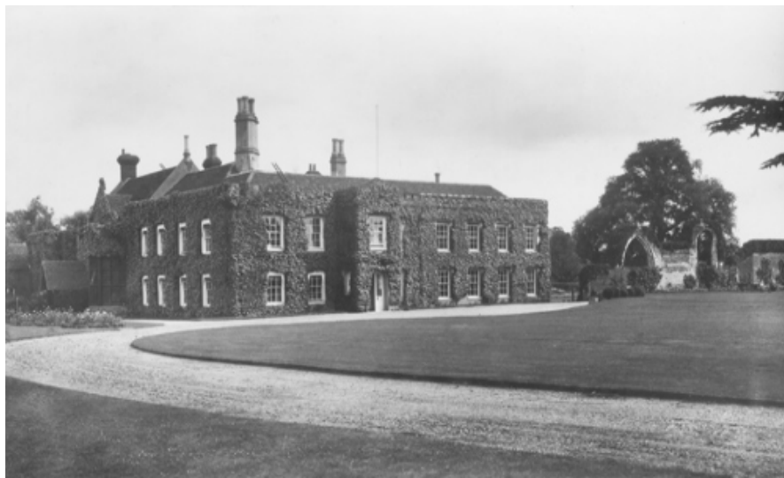
Figure 11. Circa 1950 photograph of Thoby Priory House. Priory Ruins on right. (LostHeritage.Org.UK)
