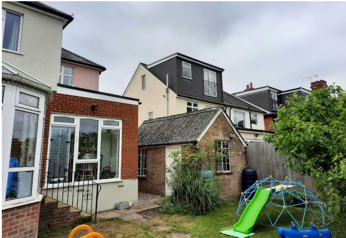
Photo above is of application house rear elevation. No. 201 in background
