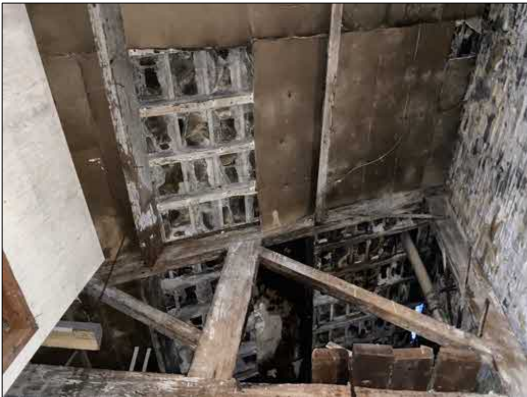
Fig 2: An internal view of the lower floor within the target building. The lower floor features extensive fire damage to the ceiling (circled).
