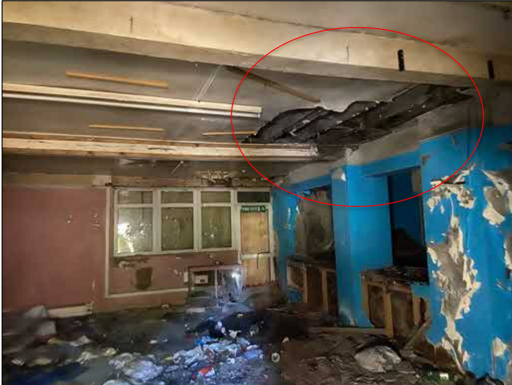
Fig 2: An internal view of the lower floor within the target building. The lower floor features extensive fire damage to the ceiling (circled).
