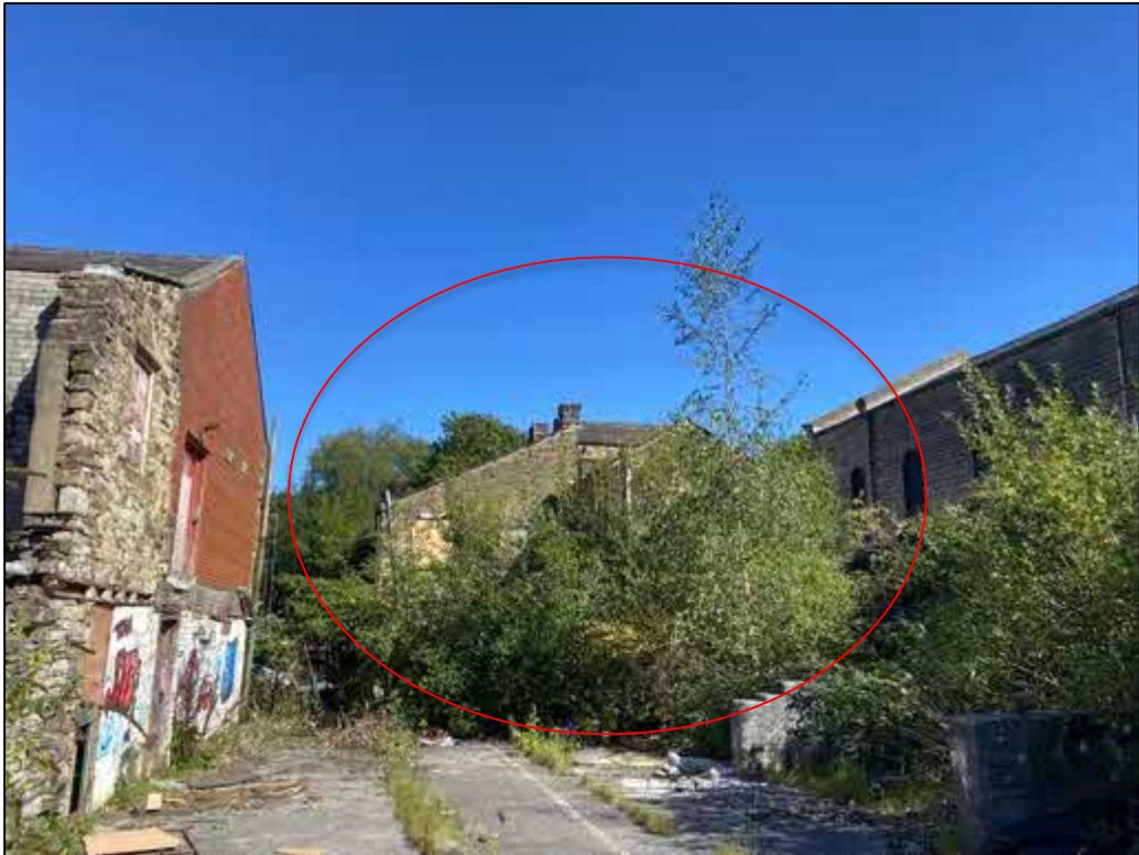
Fig 5: A rear view of the subject building. The building features several differing roof sections and smaller chimneys.
