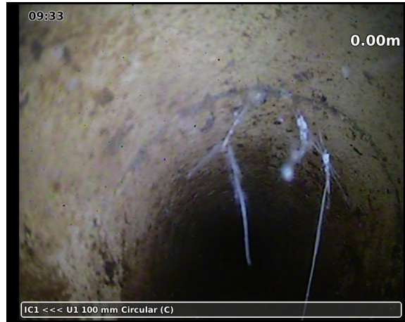
20230328-093329-snap0001.jpg, 00:00:06, 0.00 m Water level, 0% of the height
