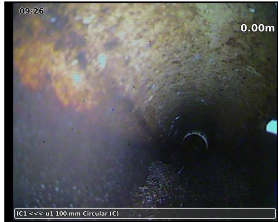
20230328-092631-snap0001.jpg, 00:00:04, 0.00 m Water level, 0% of the height
