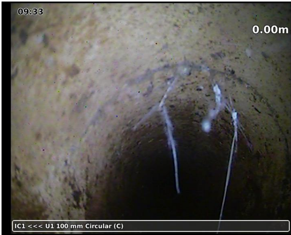
20230328-093329-snap0000.jpg, 00:00:04, 0.00 m Start inspection chamber
