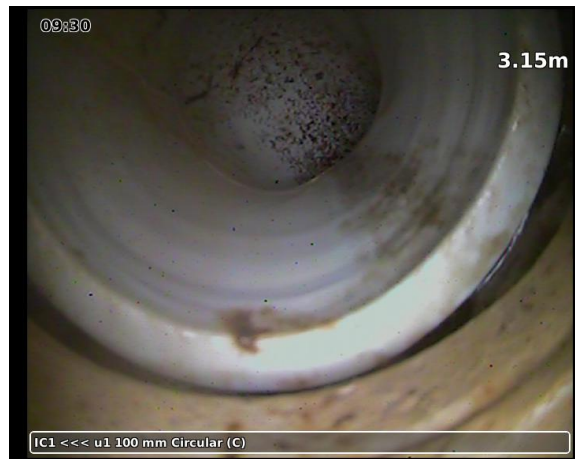
20230328-092631-snap0007.jpg, 00:04:21, 3.15 m Medium open joint
