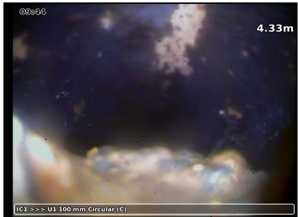
IC1X_25435ae2-dceb-4ab0-8dd4-7d4206f49c7d_20230403_1 00133_106.jpg, 00:02:37, 4.33 m Fine settled deposits, 30% area loss
