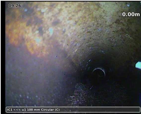
20230328-092631-snap0000.jpg, 00:00:02, 0.00 m Start inspection chamber
