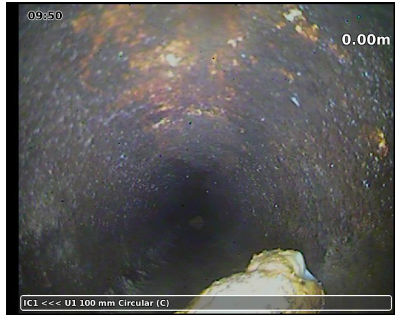
20230328-095032-snap0001.jpg, 00:00:10, 0.00 m Water level, 0% of the height
