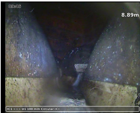
20230328-094135-snap0008.jpg, 00:05:04, 8.89 m Finish inspection chamber
