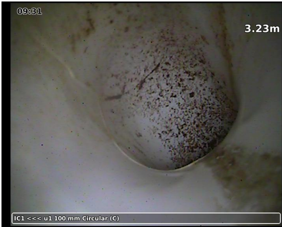
20230328-092631-snap0008.jpg, 00:05:02, 3.23 m Finish connection without manhole
