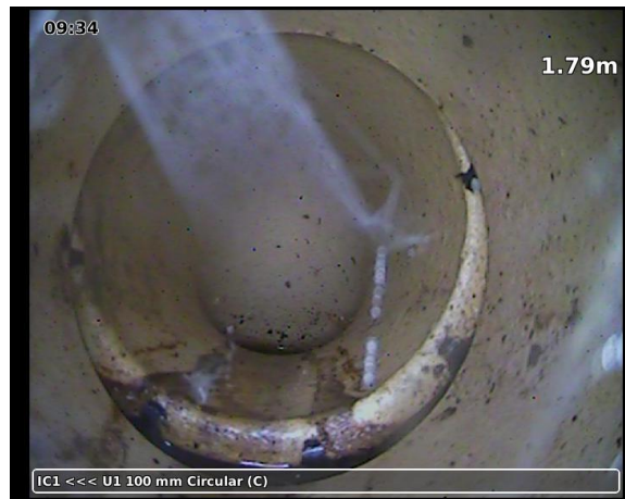
20230328-093329-snap0003.jpg, 00:00:54, 1.79 m Medium open joint
