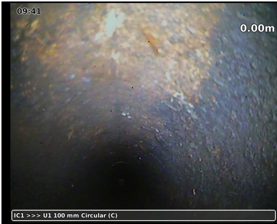
20230328-094135-snap0000.jpg, 00:00:03, 0.00 m Start inspection chamber
