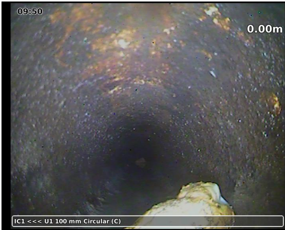
20230328-095032-snap0000.jpg, 00:00:06, 0.00 m Start inspection chamber
