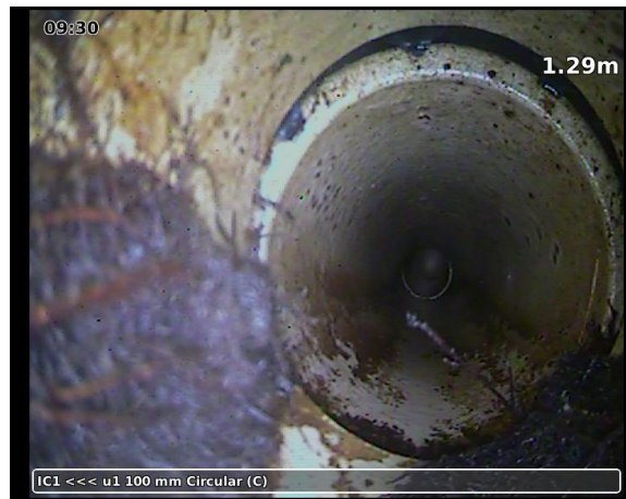
20230328-092631-snap0003.jpg, 00:03:27, 1.29 m Large open joint
