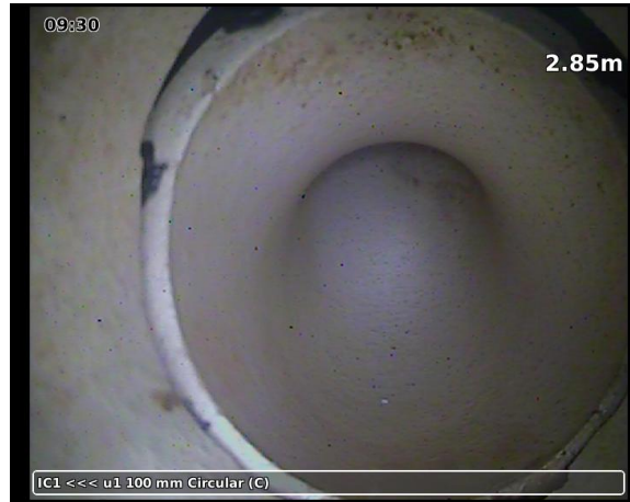
20230328-092631-snap0005.jpg, 00:04:02, 2.85 m Medium open joint
