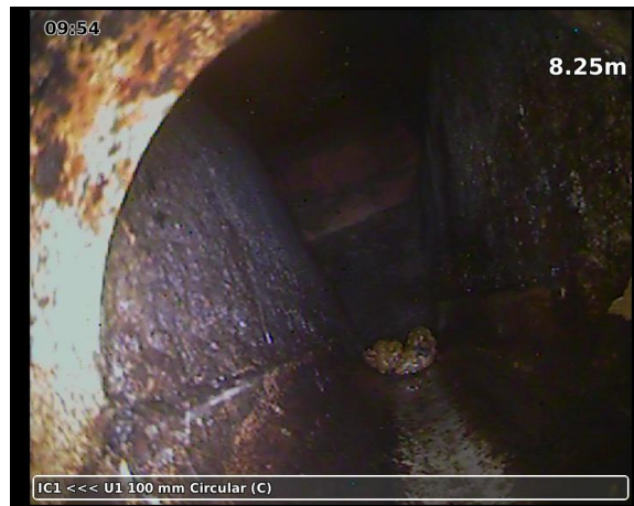
20230328-095032-snap0003.jpg, 00:04:05, 8.25 m Finish inspection chamber
