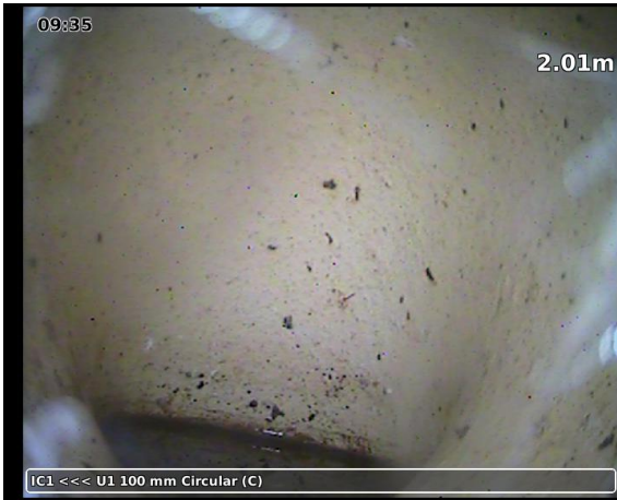
20230328-093329-snap0004.jpg, 00:01:30, 2.01 m Finish connection without manhole
