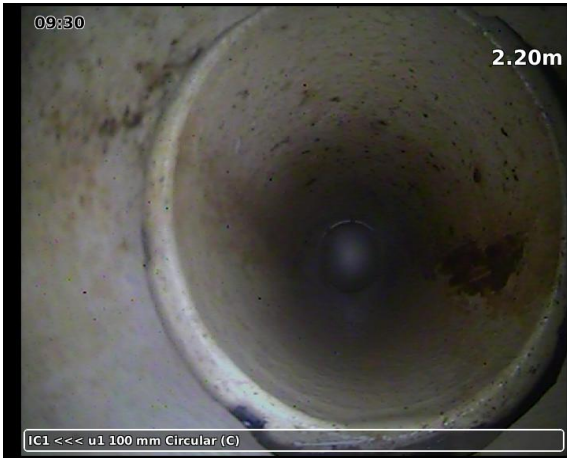
20230328-092631-snap0004.jpg, 00:03:51, 2.20 m Medium open joint
