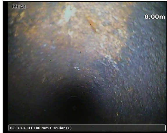
20230328-094135-snap0001.jpg, 00:00:06, 0.00 m Water level, 0% of the height
