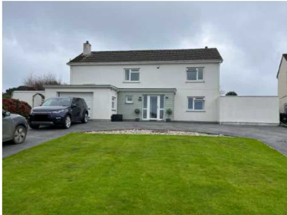
Photograph 1. Front (north) elevation.
