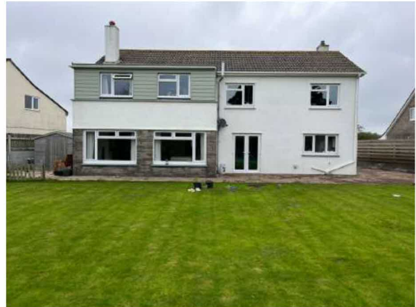
Photograph 2. Rear (south) elevation.
