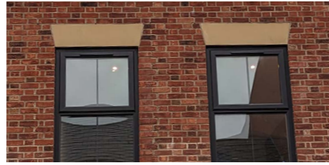
Sandstone Window Headers
