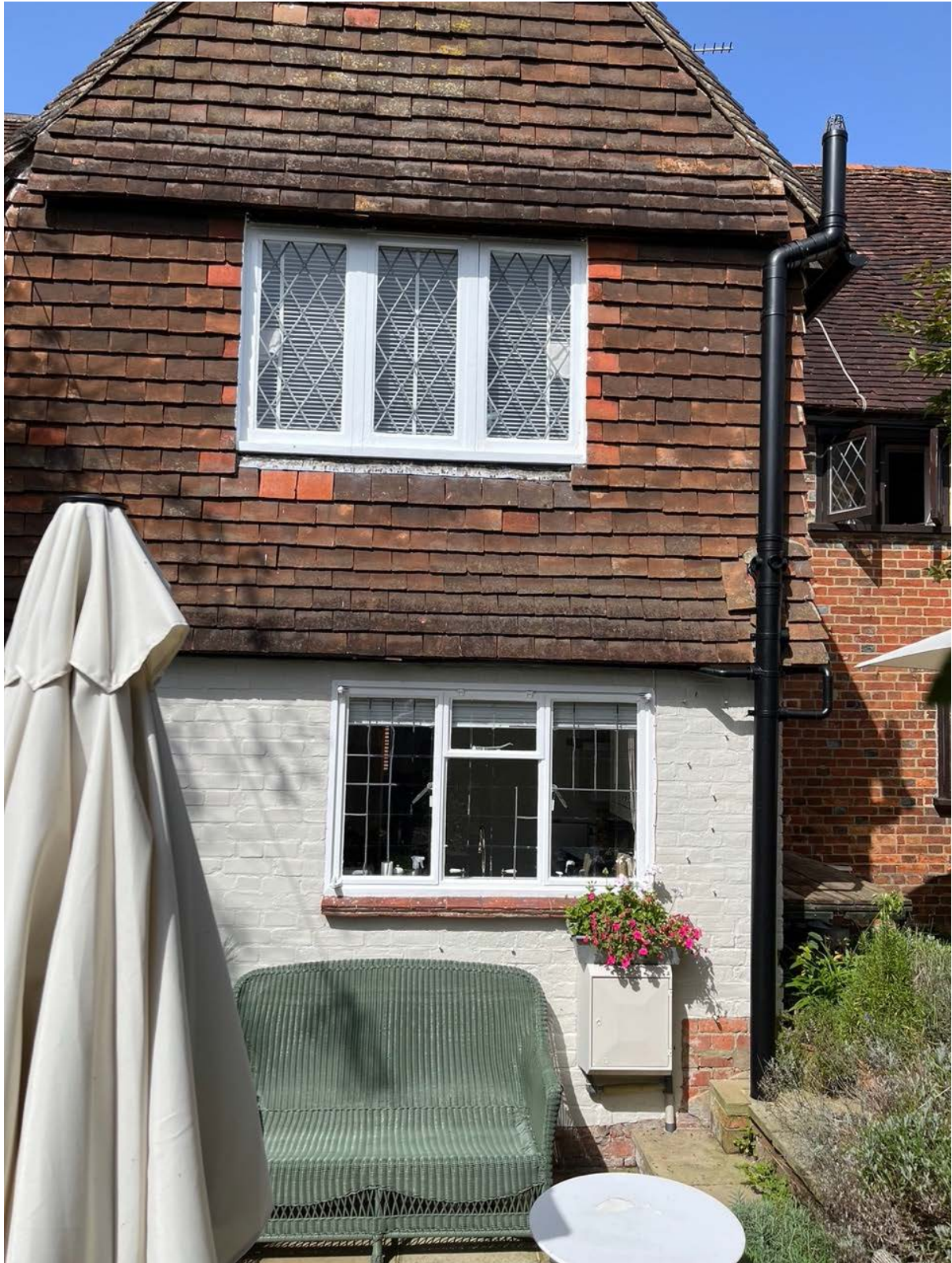
Photograph of the rear showing the two storey gable containing the two windows proposed to be replaced.
