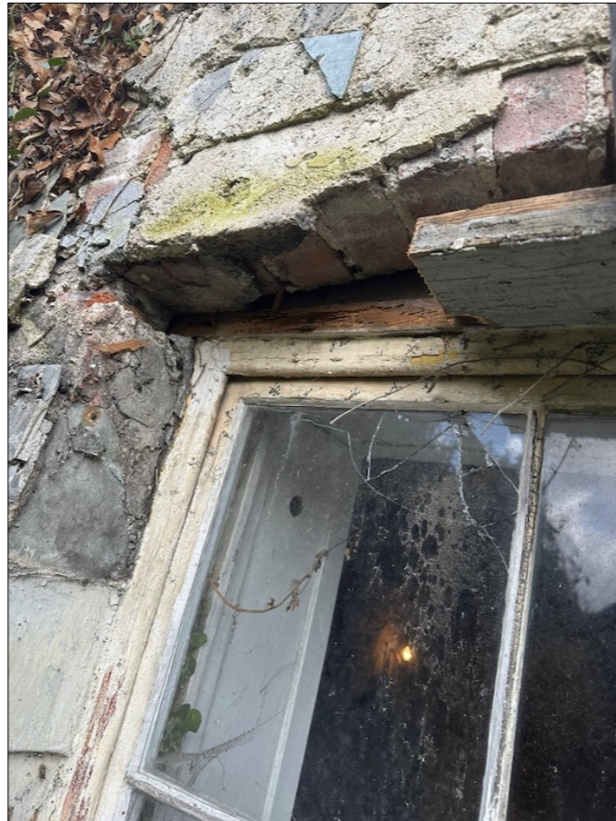
There are signs of previous repairs to sills, stiles, and meeting rails
