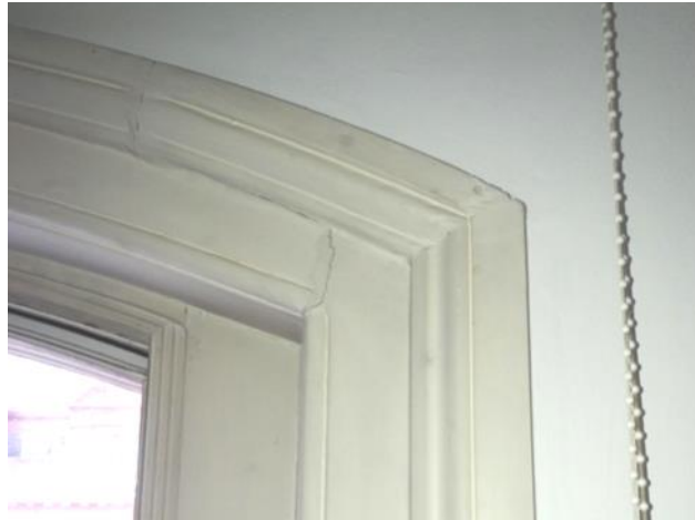
Figure 5.23: Showing the window architrave.
