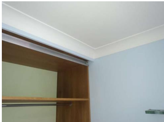
Figure 5.33: Showing the coving in the room.
