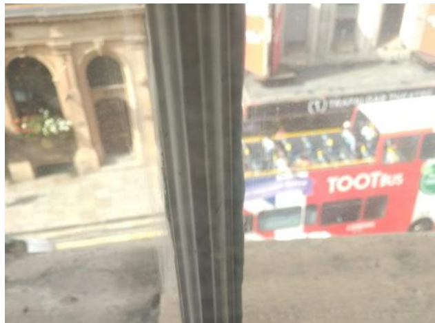
Figure 5.25: Showing the central glazing bar of the sitting room window.
