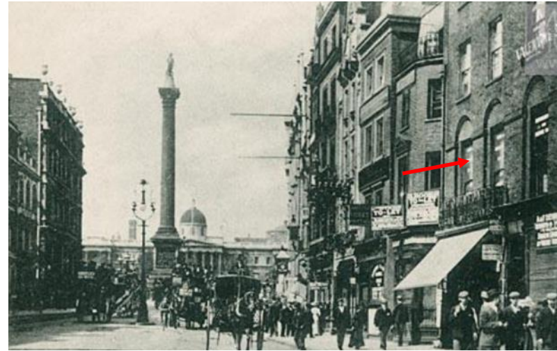
Figure 5.2: 1910 photograph looking towards Nelson's Column. No. 25 Whitehall marked in red (Source: Historic England Archives).
