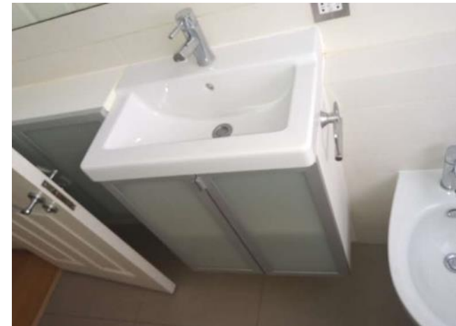
Figure 5.38: Showing the modern fittings in the Eastern Bathroom.
