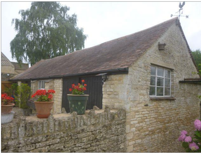
Plate 1: View of the East and North Elevation of the Barn
