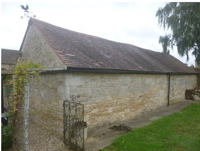
Plate 2: View of the West Elevation of the Barn
