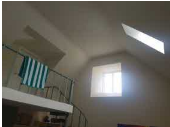
Photo 8: B2 – Internal view.
