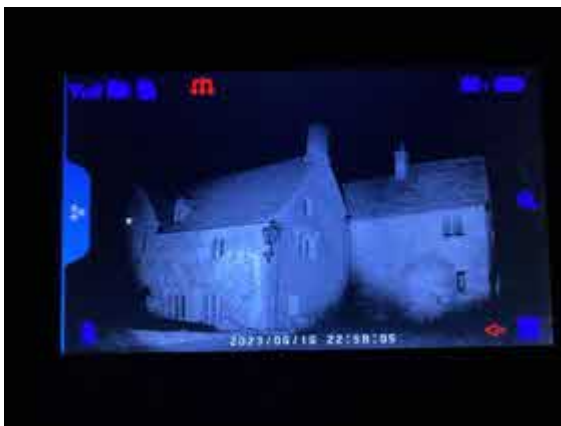
Photo 9: Example infrared camera view – east facing elevations B1.
