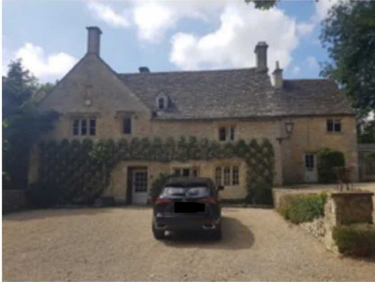
Photo 1: B1 - NE facing elevations.
