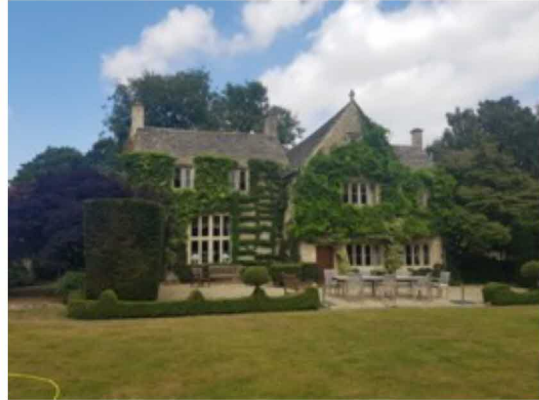
Photo 2: B1 - SE facing elevations.
