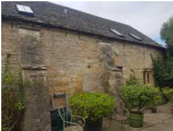
Photo 7: B2 - NE facing elevation.
