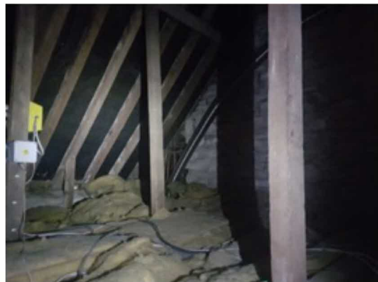
Photo 6: B1 - Internal view of loft void 2.
