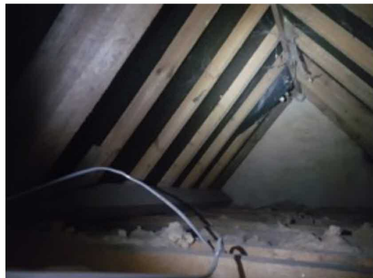
Photo 4: B1 - Internal view of loft void 1.
