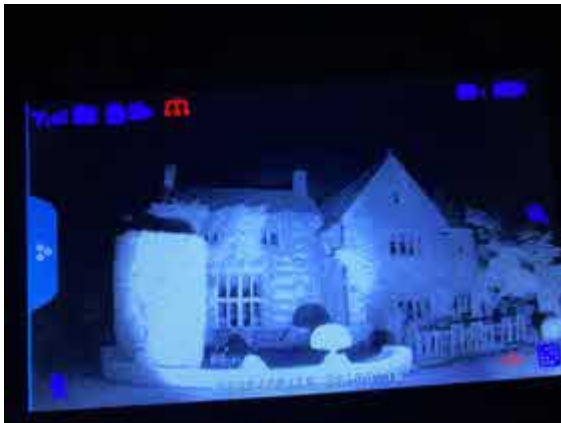
Photo 11: Example infrared camera view – south-facing elevation B1.
