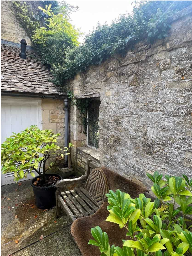
Image above: photo showing the rear, north (courtyard) side of the connecting wall. Note the more random rubble stonework, different to the S side.
