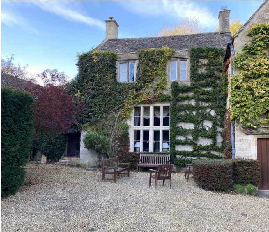
Image above: photo showing the south elevation of the early / mid C17 phase. The double height mullion window has a fine double ovolo moulding whilst the 1F window is only single. The double ovolo moulding is seen at Rectory Farm in Turkdean and is mid C17. It is thought the same mason worked on both these buildings consecutively.
