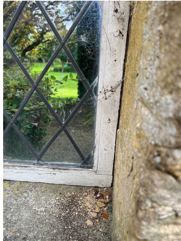
Image above: photo showing infilled opening, undertaken by Alan Mansfield Smith in the 1950s. Note the lead is clipped short and the beading is tacked on, clearly C20.
