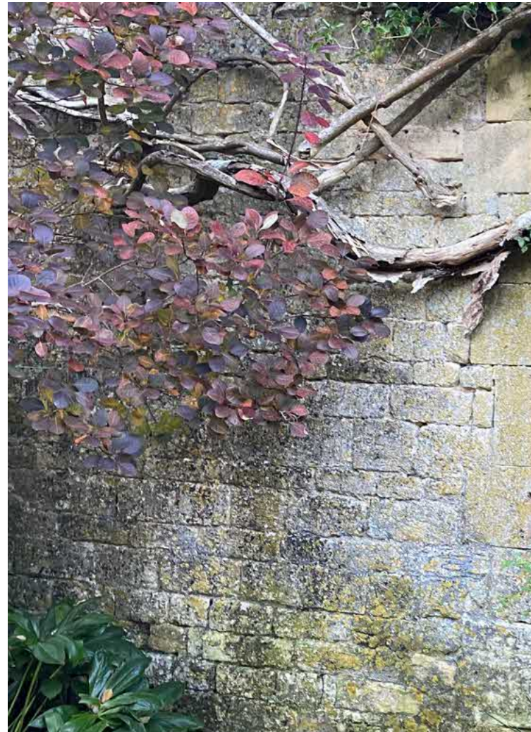
Image above: photo showing south (lawn) side of wall, with coursed and square faced stonework which appears C19 in origin.
