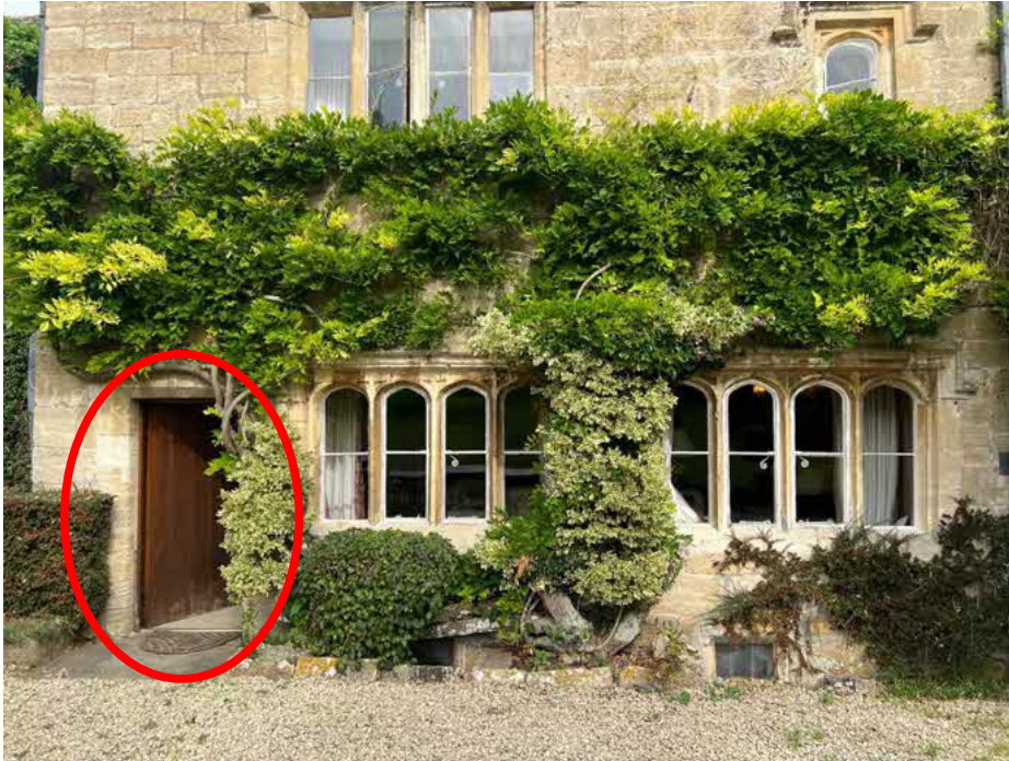
Image above: photo showing south elevation of main range with the modern door, in the historic opening from where the garden wall door was taken. The modern door was replaced during the 1970s phase of works as the older door allowed rain ingress.
