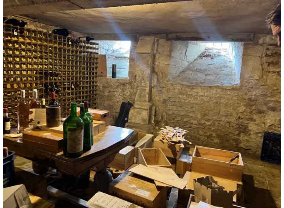
Image above: photo showing the fine buttressed cellar.
