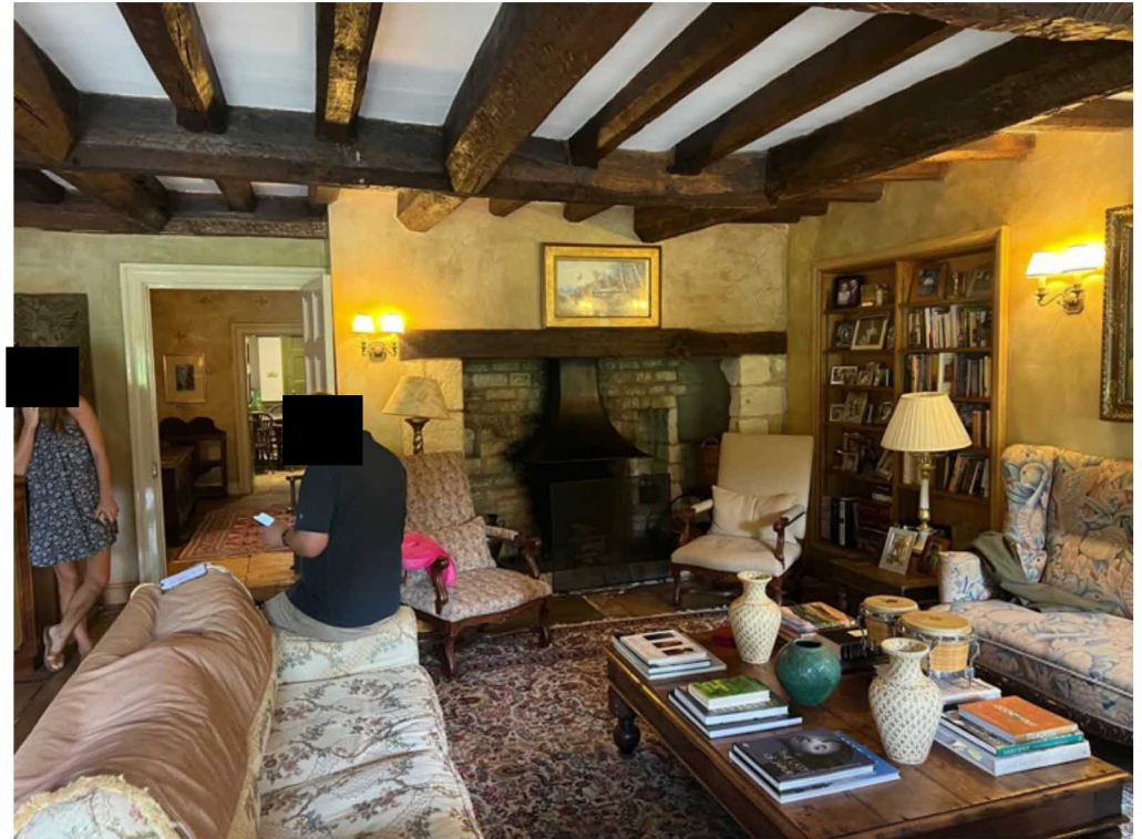
Image above: photo showing the same joists on the RHS. Note the fireplace is entirely modern.
