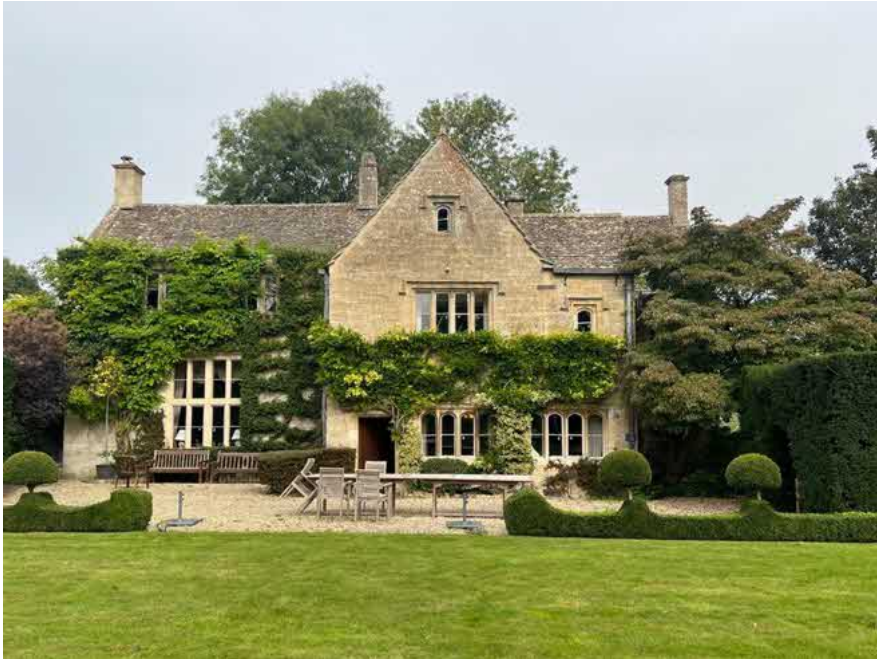
Image above: photo showing the front south elevation. The late C16 / early C17 phase is on the RHS. Note the lack of a break line in the masonry between this S front gable and the SE nose return, see below commentary .
