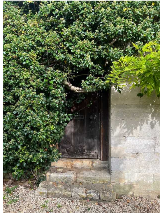
Image above: photo showing partial view of the older original door which belonged to the front door to the east of this. The frame is modern; the door allowed rain ingress and hence new frame.
