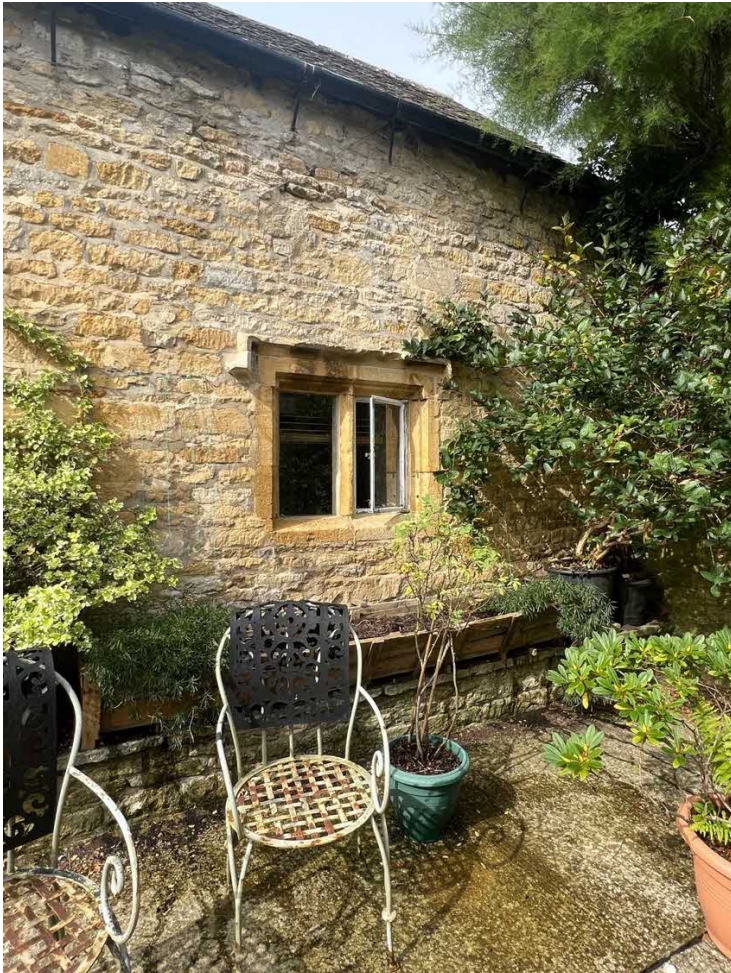
Image above: photo showing mullion window of C17 barn.
