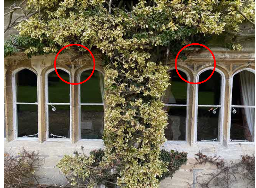
Image above: photo showing the 2 4-light mullions on the front elevation. Note the different spandrel details to the lancet heads. It is thought the RHS window was taken from Rectory Farm, in Turkdean.
