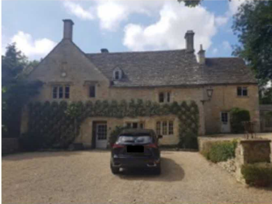
Photo 1: B1 - NE facing elevations.
