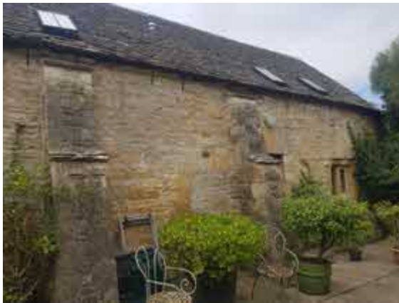
Photo 7: B2 - NE facing elevation.
