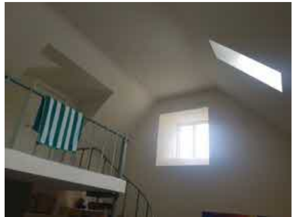
Photo 8: B2 – Internal view.
