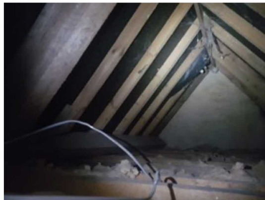
Photo 4: B1 - Internal view of loft void 1.
