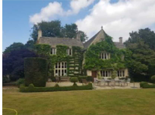
Photo 2: B1 - SE facing elevations.
