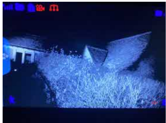
Photo 12: Example infrared camera view – south-western roof aspect B2.
