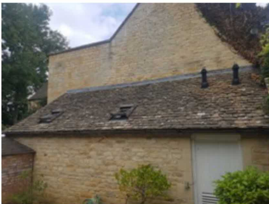
Photo 5: Cotswold stone tiles cladding mono-pitched roof element. B1.
