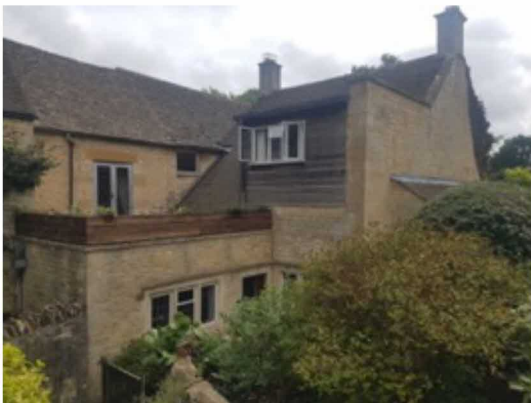
Photo 3: B1 - SW facing elevations showing flat roofed element and balcony.
