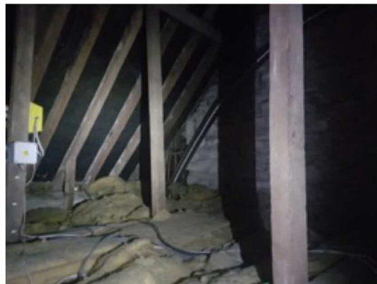
Photo 6: B1 - Internal view of loft void 2.
