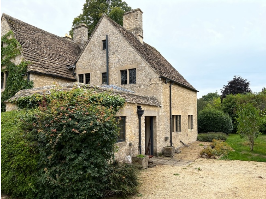
Image above showing stone-tiled parapet by Norman Jewson, early C20. The conversion behind is modern, just discernible by the roof lantern.
