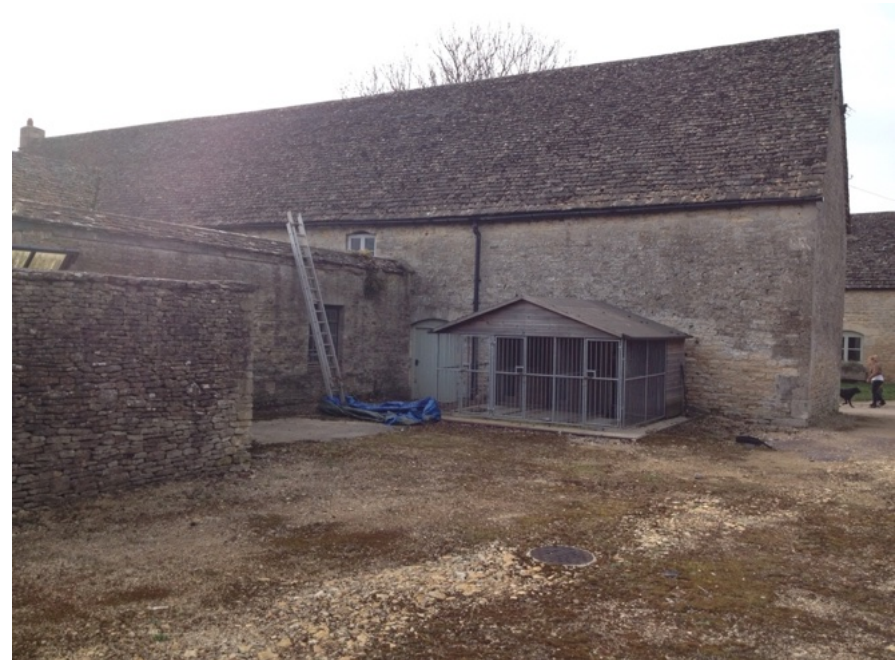
Image above showing stone-tiled parapet at a GII barn in south Cotswolds, done in the early C20, and which now hides a garage behind it.
