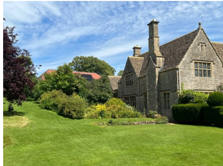
Above images showing moulded string courses on buildings by Jewson (below) and Dawber (above).
