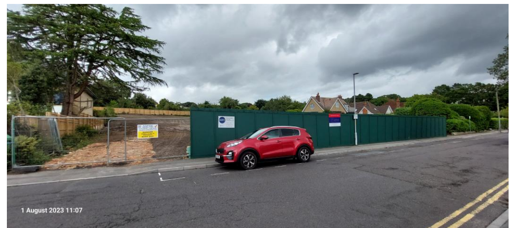
Photo 4: Southern boundary of the site.
