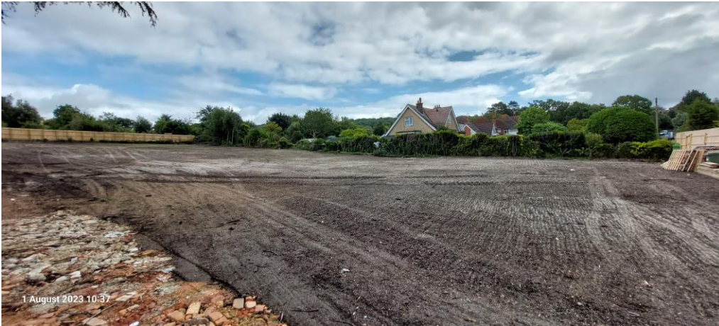
Photo 1: Cleared site showing bare ground.
