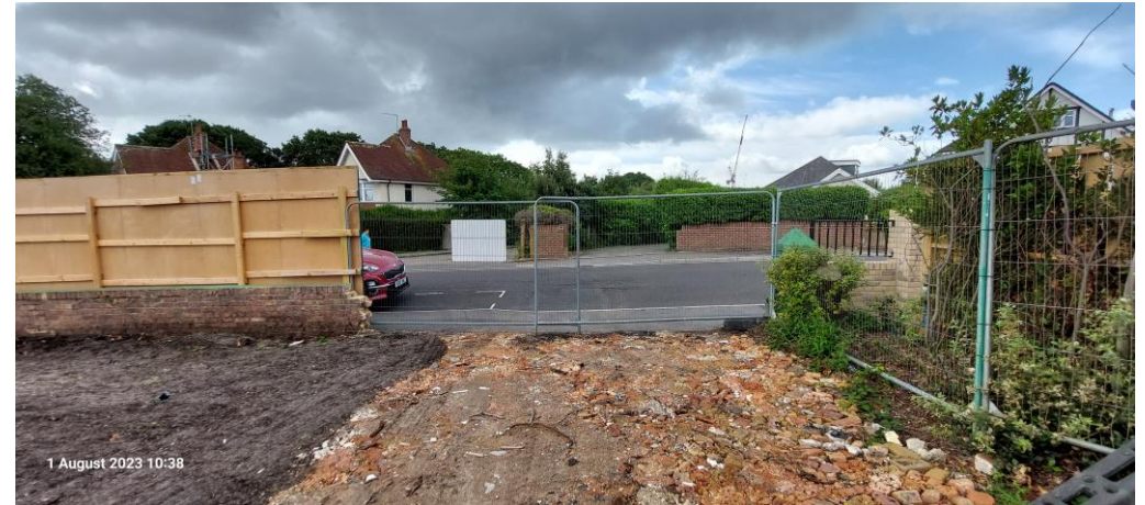
Photo 2: Southern access to the site.
