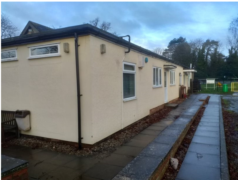
Village Hall eastern elevation
