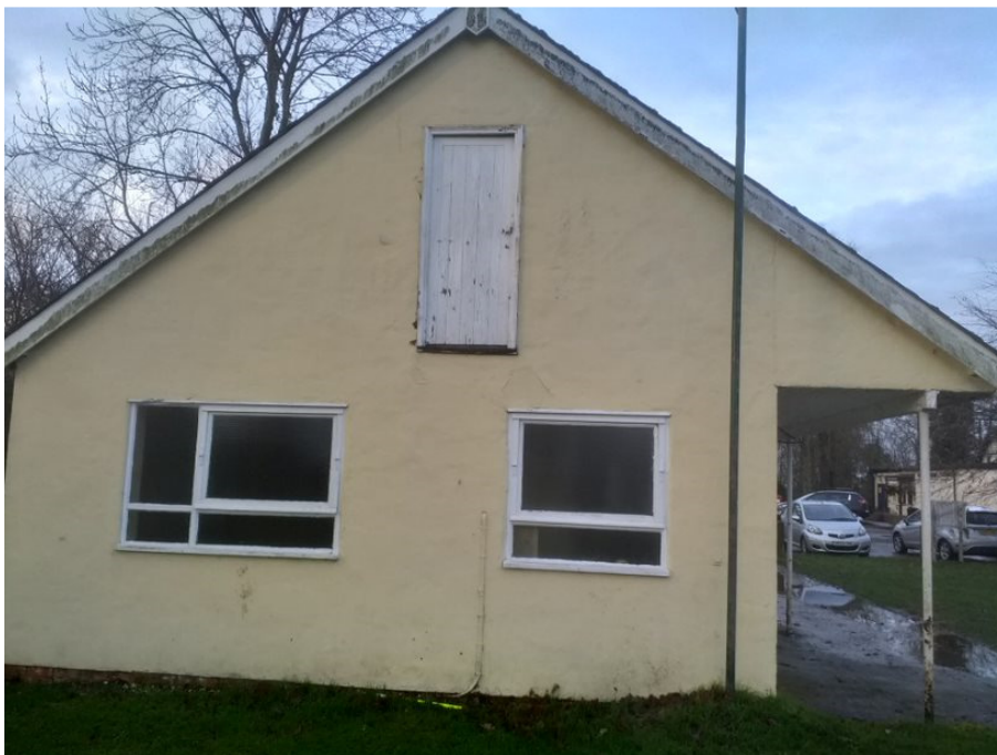
Eastern elevation of pavilion. Note entry door into roof void
