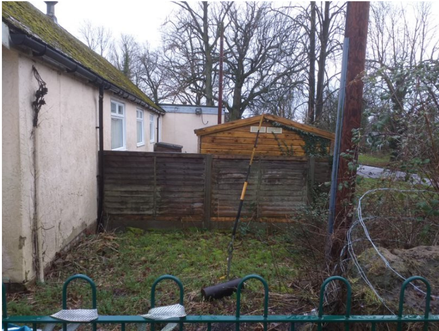
Western side of hall
