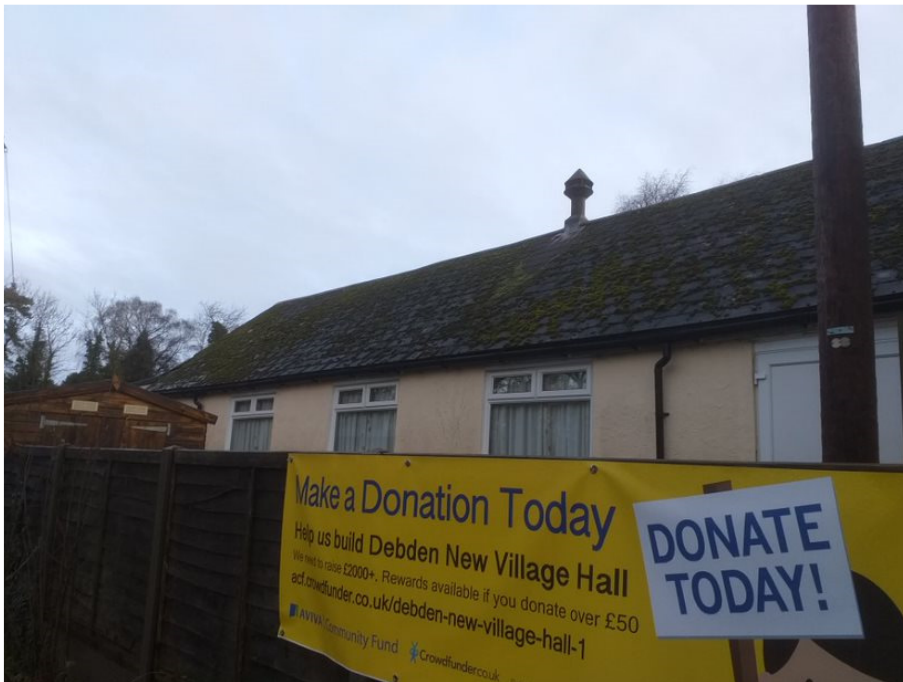
Village Hall western elevation
