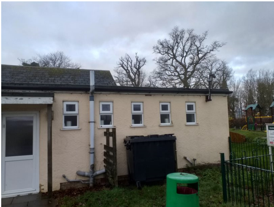
North eastern elevation of hall
