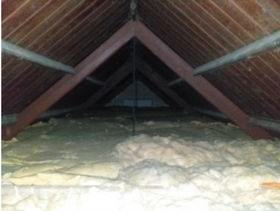
Roof void above hall. No evidence of bats
