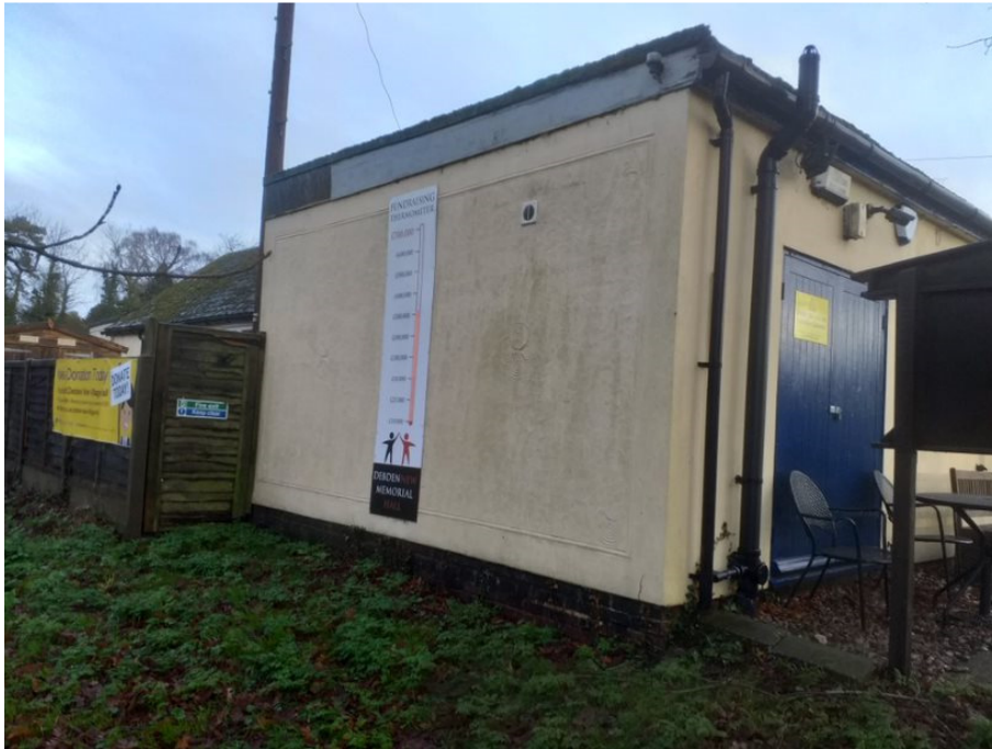
Village Hall / shop south western elevation
