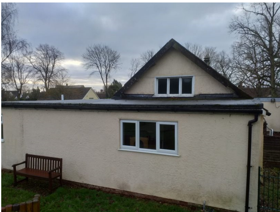
Northern elevation of hall
