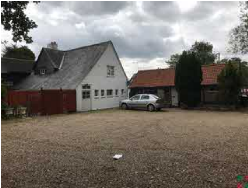
Photograph 4 Looking south from the restaurant car park to the rear of the restaurant building.
