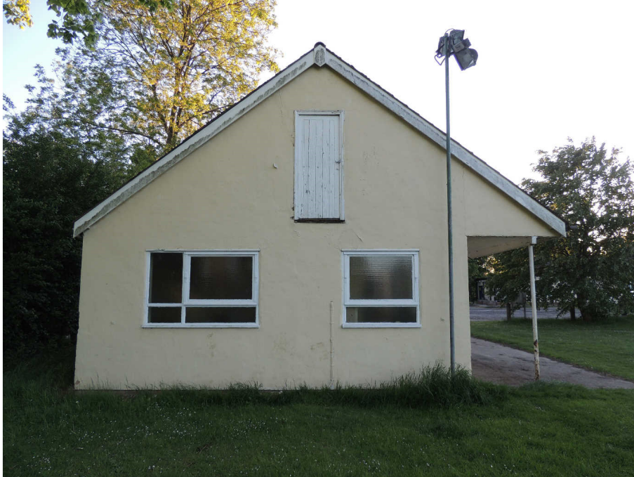
Photo 3: Eastern elevation. The door provides access to the loft
