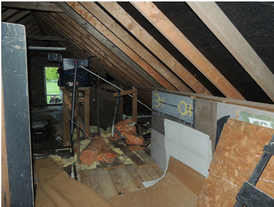
Photo 6: Looking eastwards in loft
