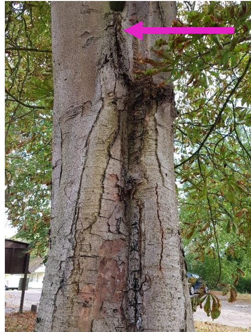
Photo 9 of T19 tight fork. A climbing inspection is recommended to probe the union, with a view of bracing or reducing the crown.
