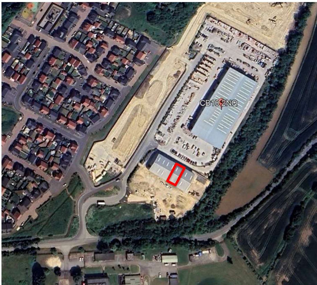
Aerial view of the site and surroundings, with the approximate boundaries of the application site annotated in red
