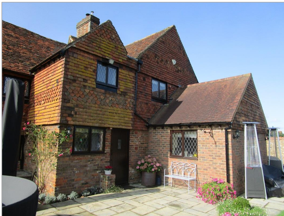
Fig. 4: The 1990 (left) and 1991 two-storey gabled additions are faced with reclaimed bricks on the ground floor and tile hung above, with alternating broad bands of rectangular and scalloped tiles; they have plain tile roofs. The 2010 addition has less well-matching brickwork, and machine-made roof tiles.
