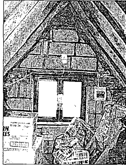
Figure 53: Northern end of roof space. Gable end wall to north elevation
