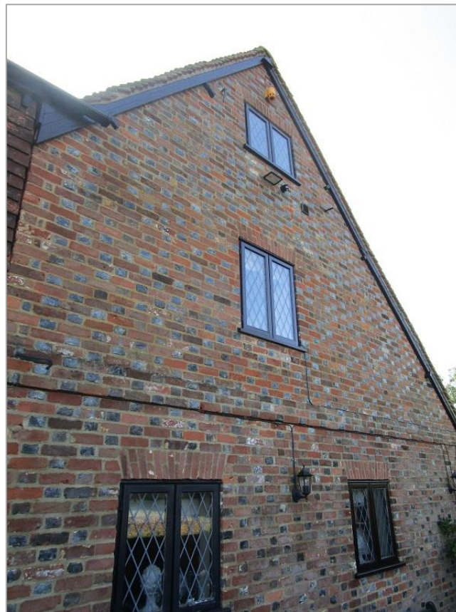
Fig. 2: North elevation of C18 north addition, in red brick with vitrified blue headers. A raised band separates the ground and first floors. The casement windows are all modern. Matching brickwork in the 1981 catslide addition to right.
