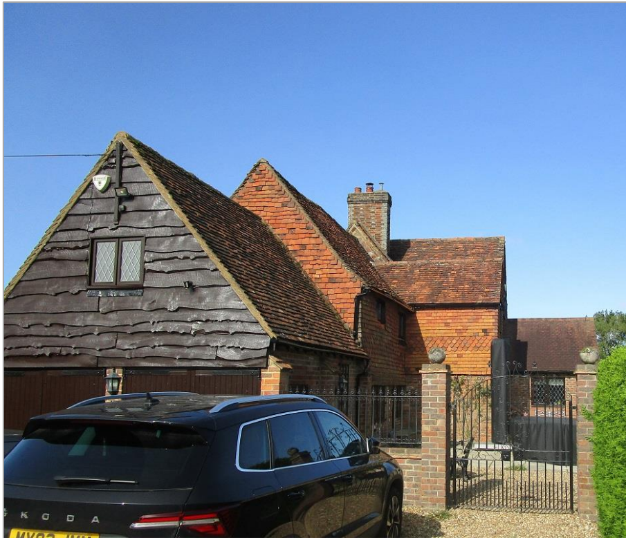
Fig. 3: The building from the south, with 1980s garage in foreground, tile hung and slightly higher original range centre, rebuilt C17 stack and higher ridge of C18 north range beyond. Giving off to the right are the lower ridge of the 1990-approved two-storey addition (attached to the original range) and the higher ridge of the 1991-approved addition (giving off the north range). To the right is the lower ridge of the 2010-approved kitchen addition.
