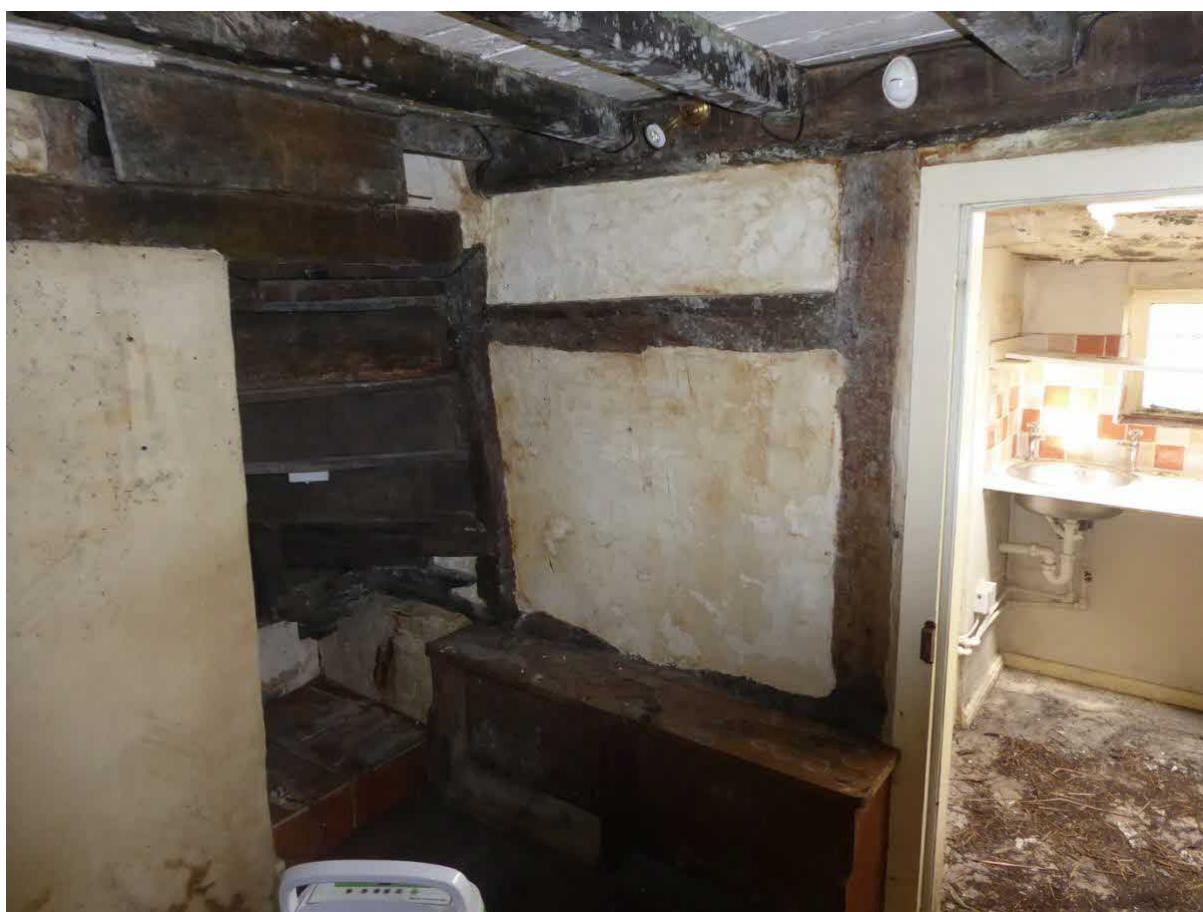
Figure 12: Lightly chamfered joists to Room G2
