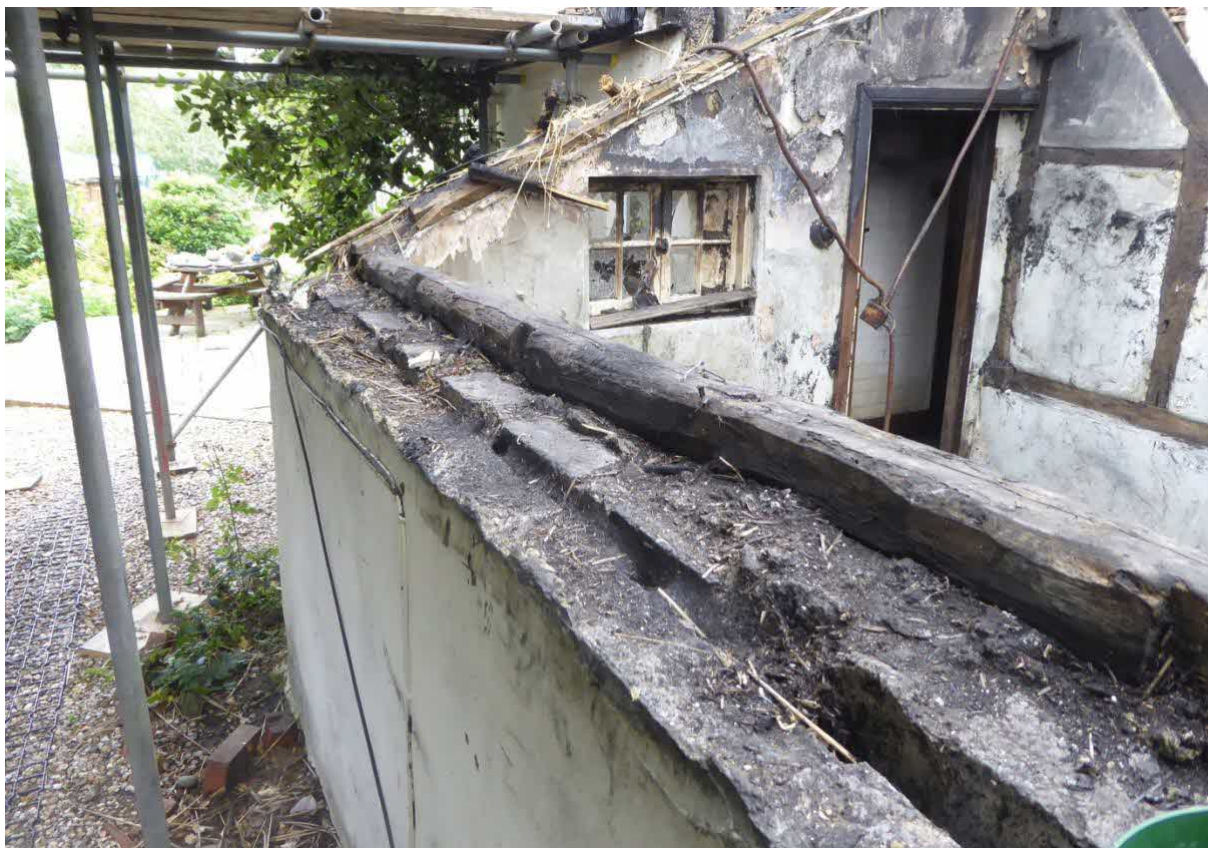
Figure 3: Cavity wall to west wall of ground floor extension to west
