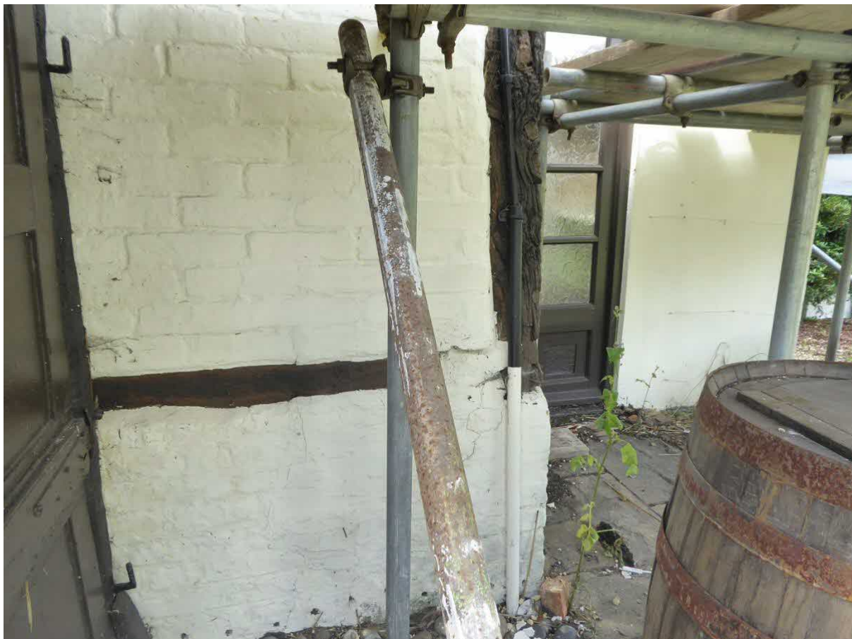
Figure 4: Mid 20 th century outshut to rear
