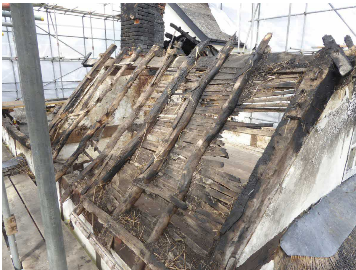
Figure 20: Room F2 -surviving section of roof
