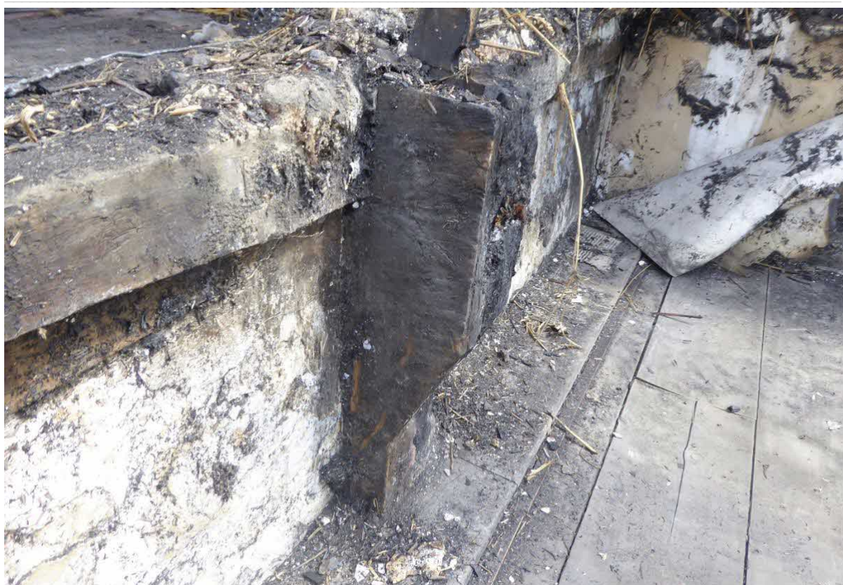
Figure 19: Jowled post to north side of Room F1
