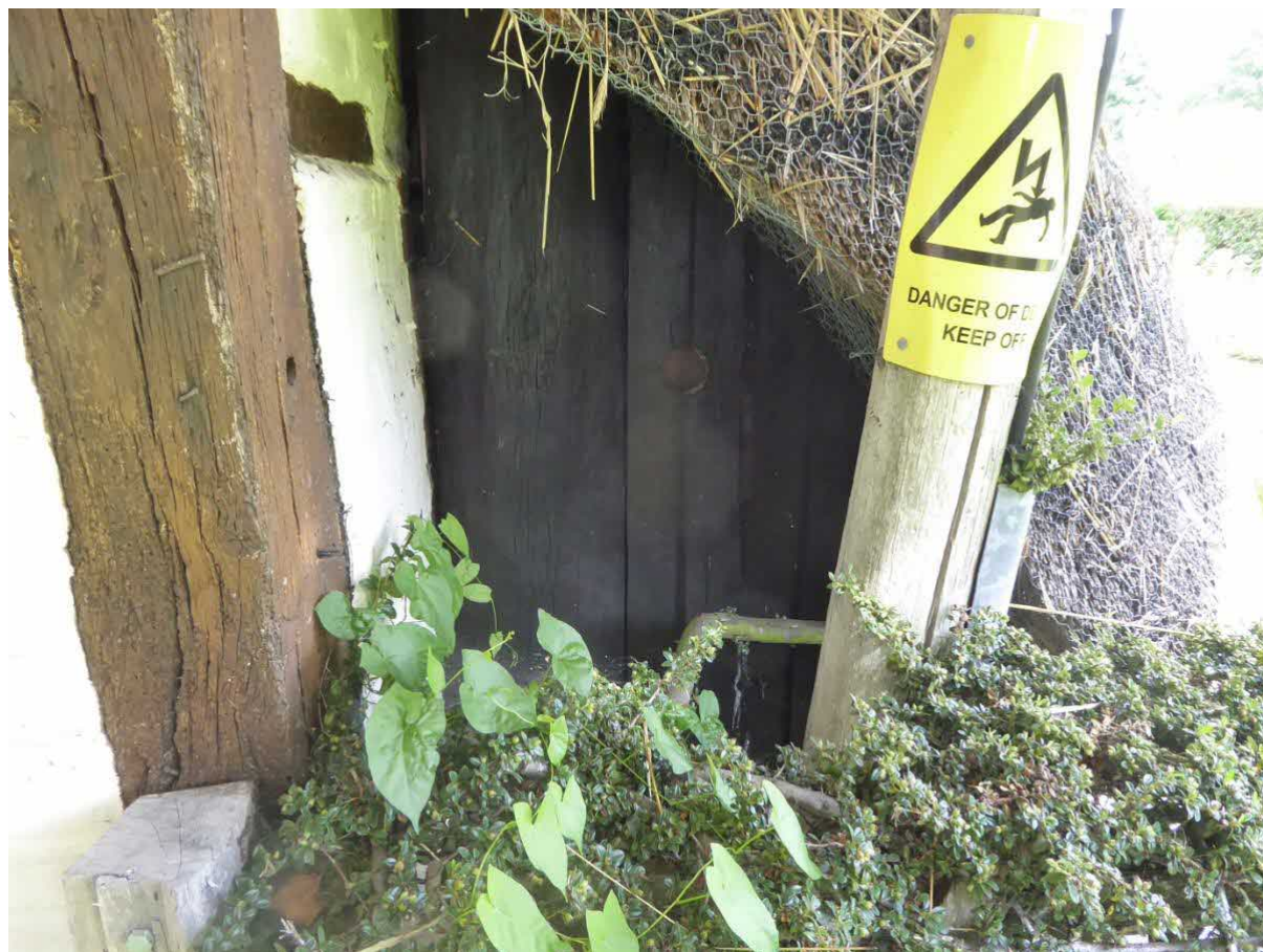
Figure 5: Store to east elevation -south side
