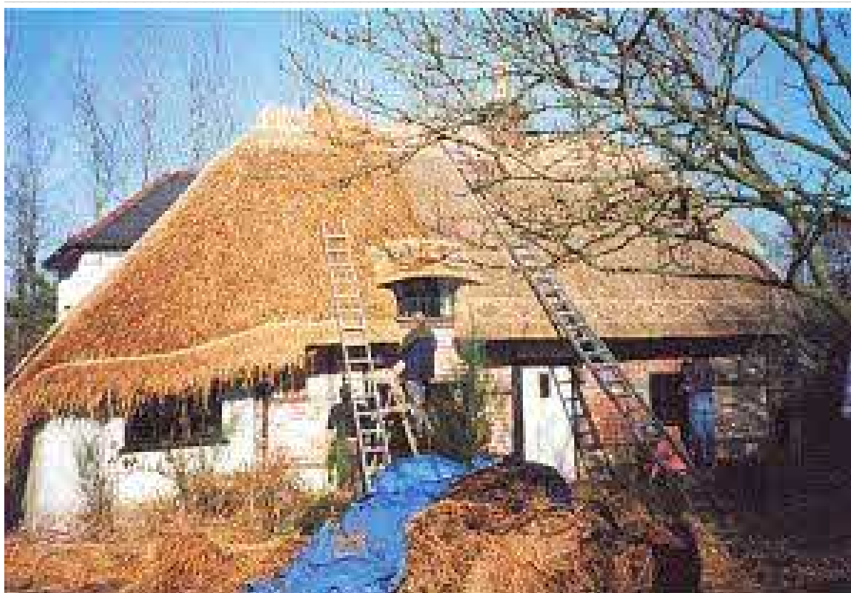
Figure HP3: Wellow Wood Cottage – post c2000 restoration during rethatching
