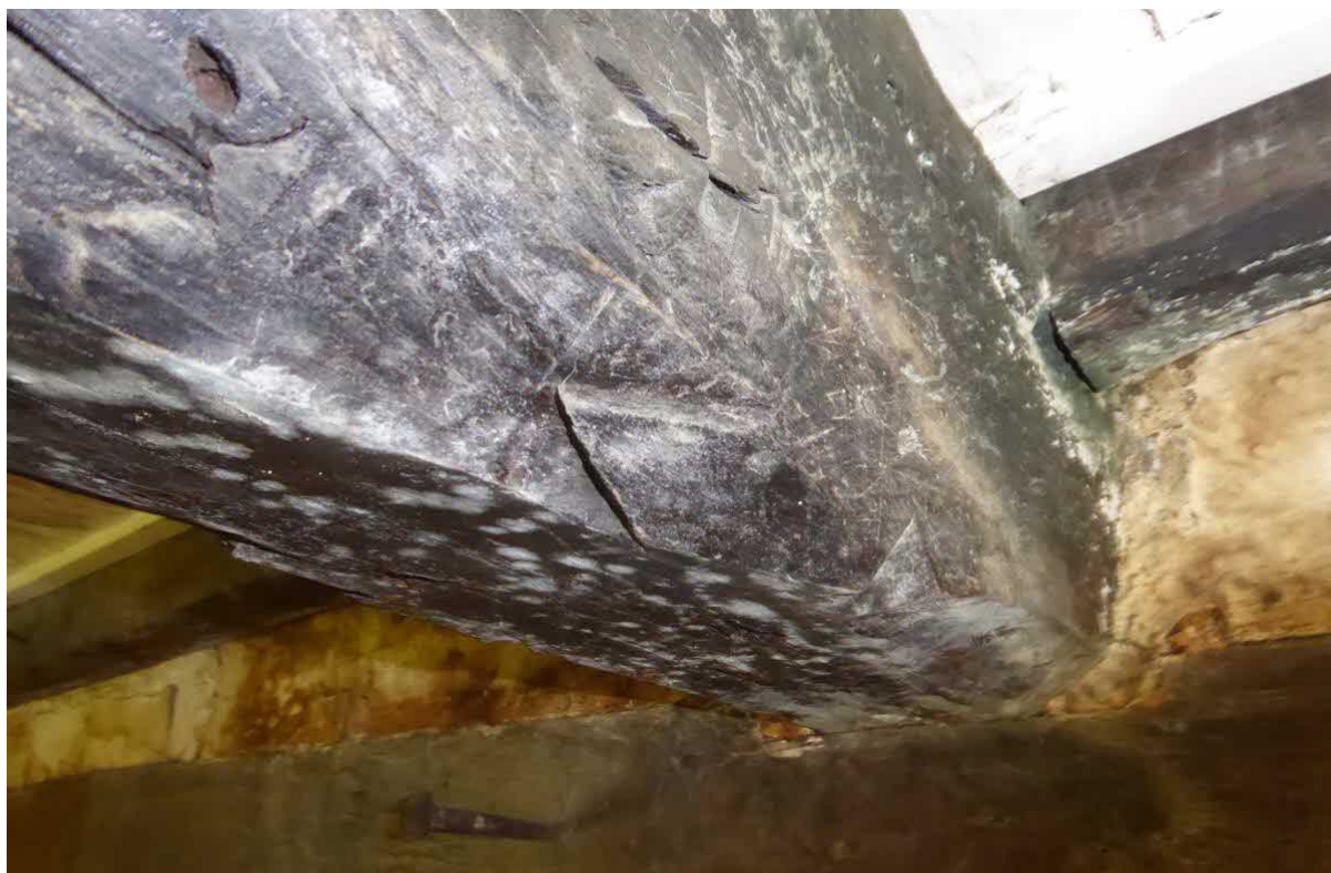
Figure 10: Chamfered stop to spine beam, Room G1 – early 17 th century
