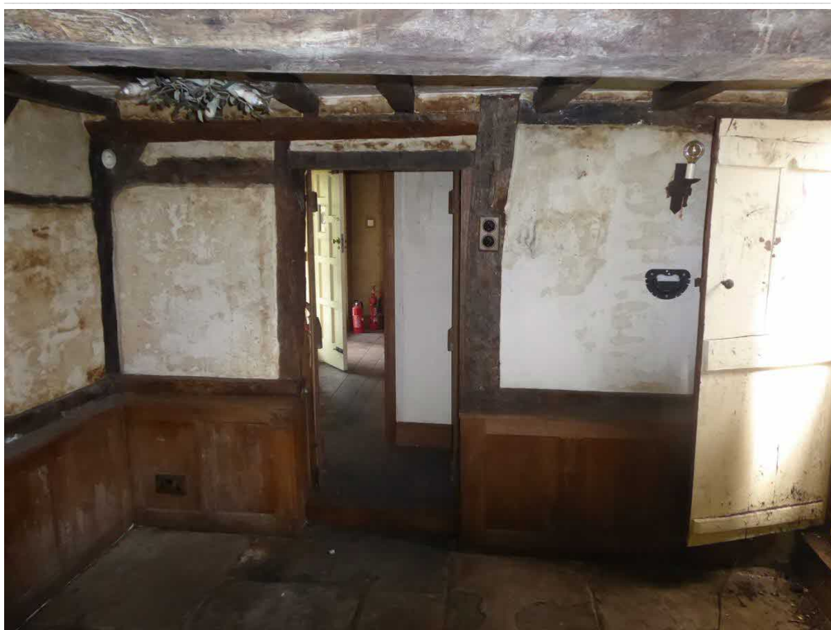
Figure 7: Oak panelling to dado rail part of c2000 'restoration'
