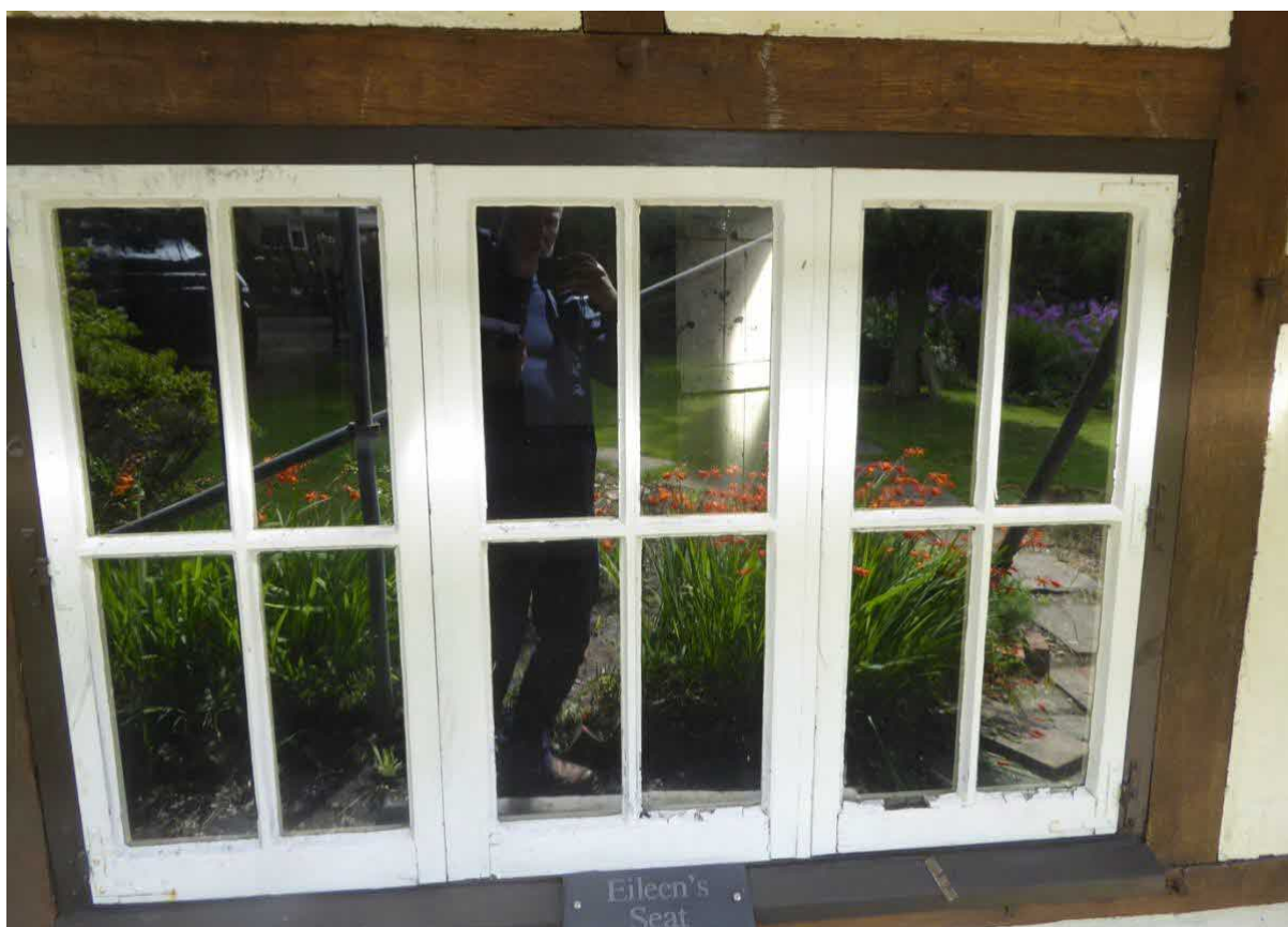
Figure 2: Window W2 – part of c2000 restoration works
