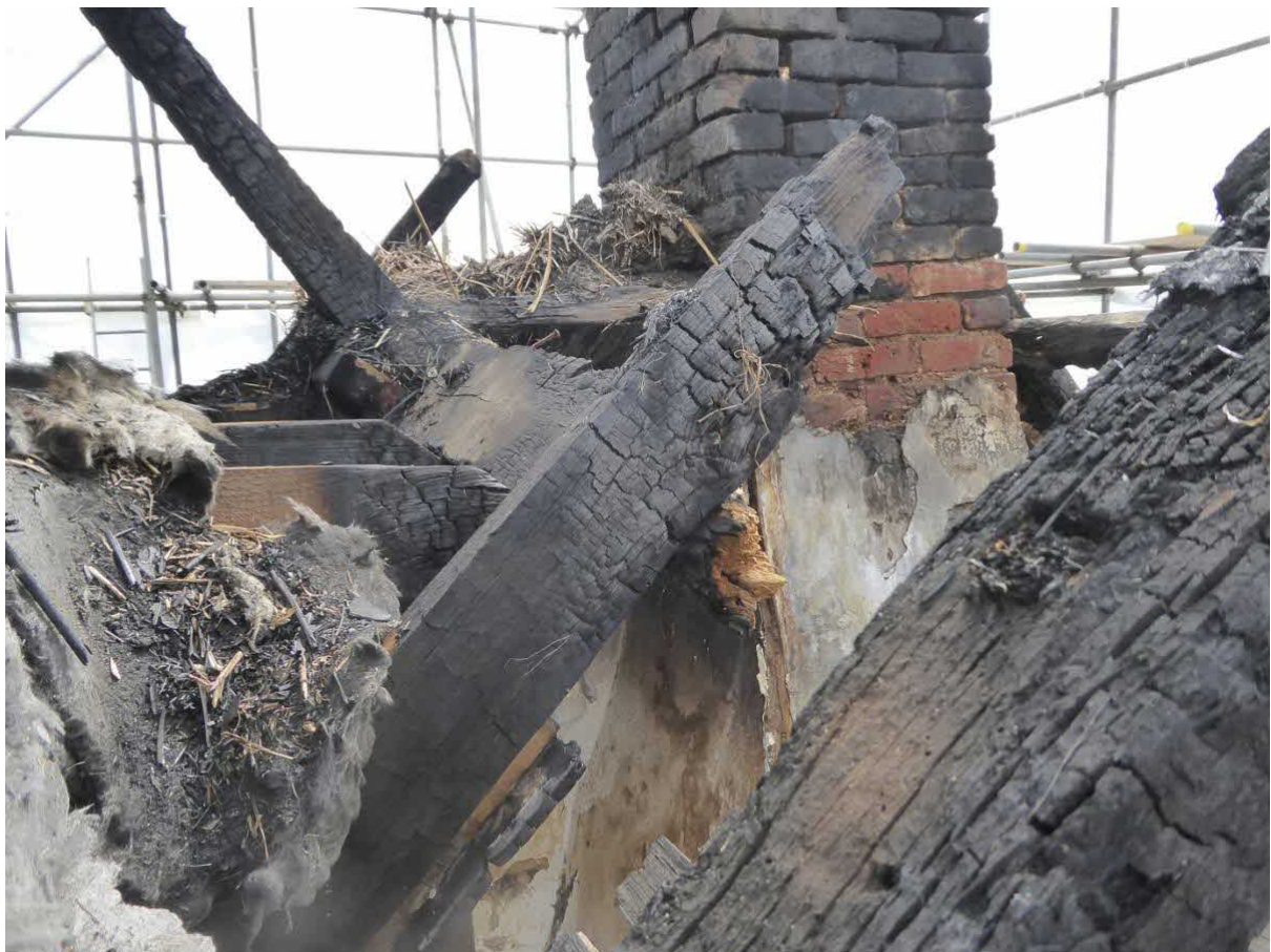
Figure 18: Small section of roof above landing/stair
