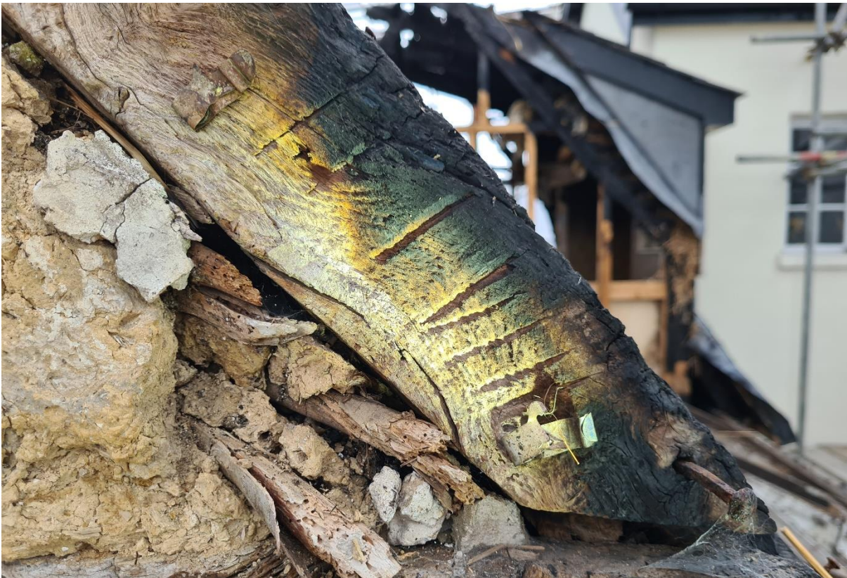
Carpenter's numerals visible at foot of principal on NE corner.
