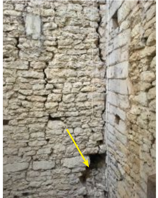
Above: South corner of the belfry/intermediate chamber with larger void visible. Below: Cracking to the belfry/intermediate walling.
