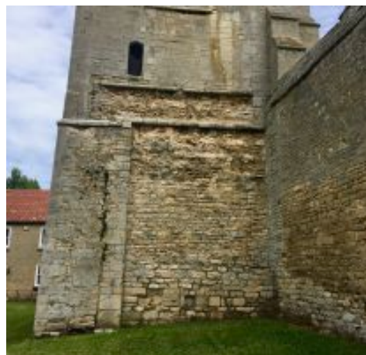
Below: Tower south elevation lower stage.
