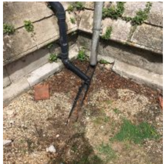
Above: RWP1 - south porch west side. Below: Base of RWP2 and RWP3 with plastic branch pipes.
