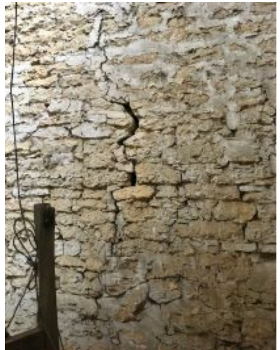
Above: South corner of the belfry/intermediate chamber with larger void visible. Below: Cracking to the belfry/intermediate walling.
