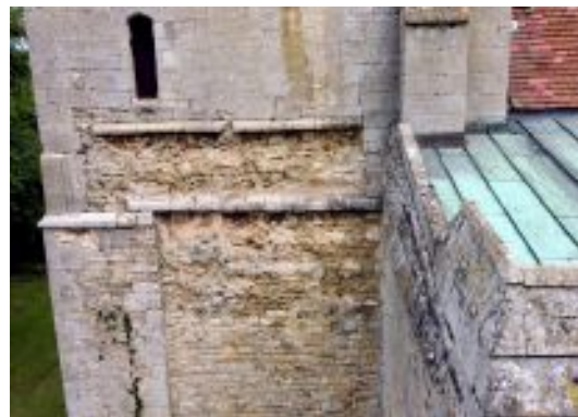
Above: Tower south elevation middle stage seen from the drone.
