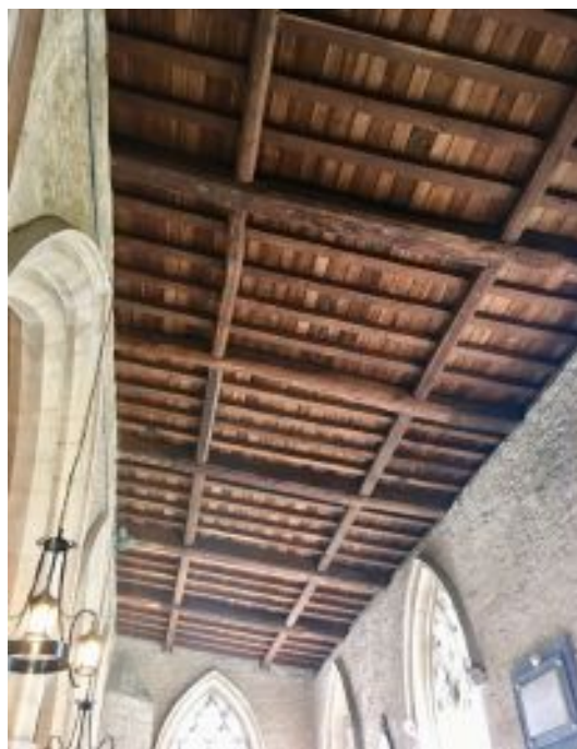
Above: Porch ceiling structure. Below: View of the south aisle ceiling.
