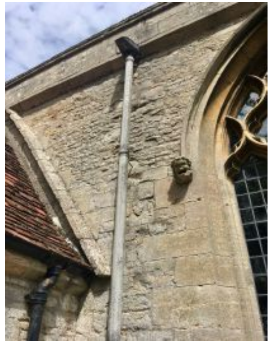
Above: RWP3 - south aisle downpipe east of the porch. Below: Base of RWP4. Bottom: RWP5 - south aisle south elevation eastern downpipe.
