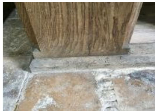
Above: Pew platform base with evidence of woodworm and death watch beetle. Below: View of the north aisle aisleway flooring.
