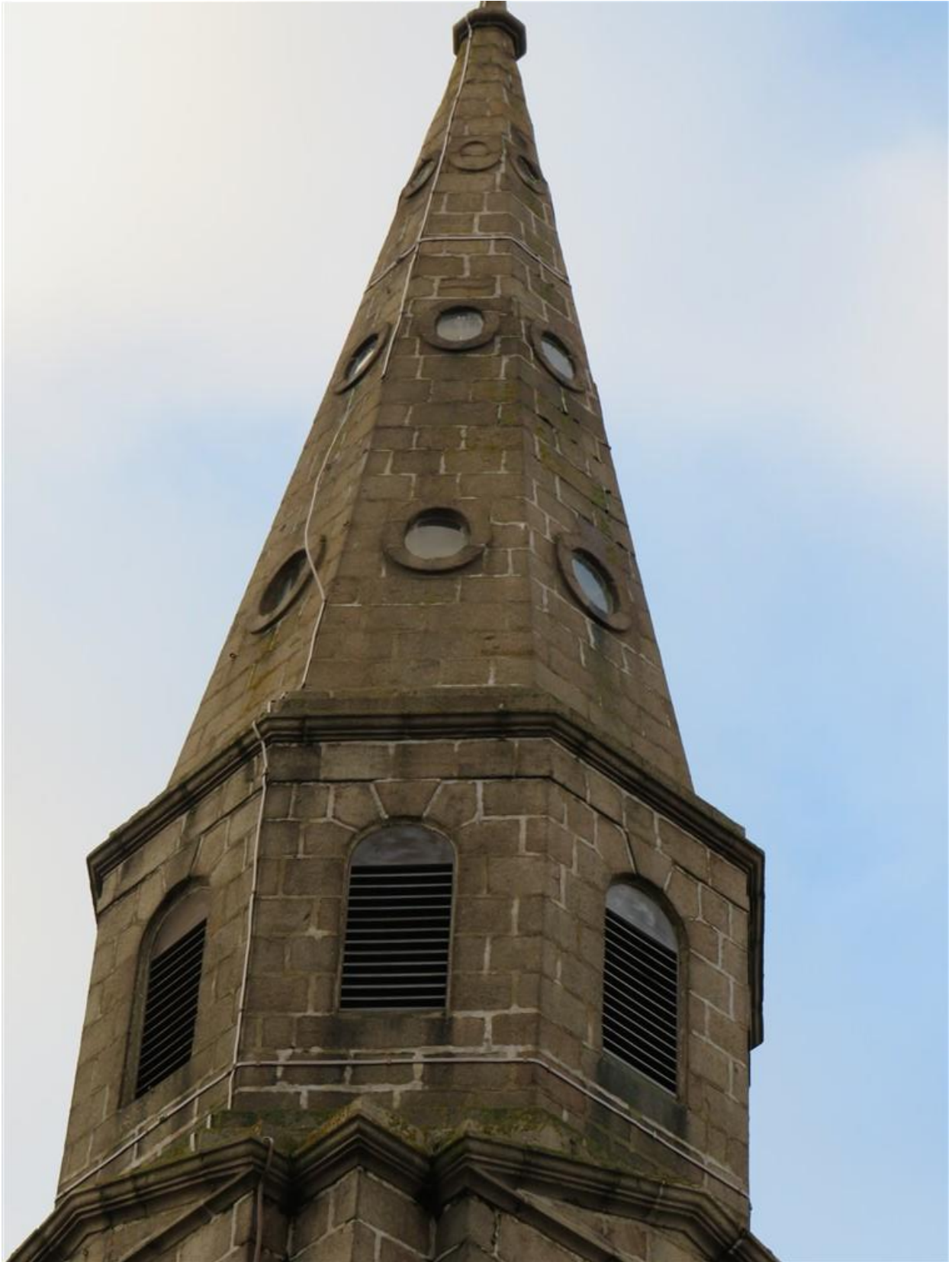
Photograph 3: Town House Bell Tower
