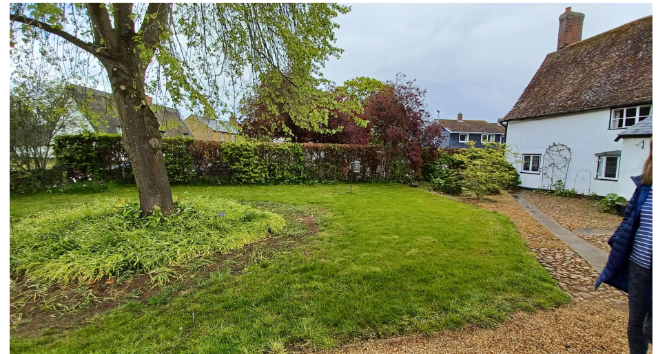
Figure 11 View across the front elevation of Kitchens Farm, looking east. This front garden is considered to contribute to the significance of the asset.
