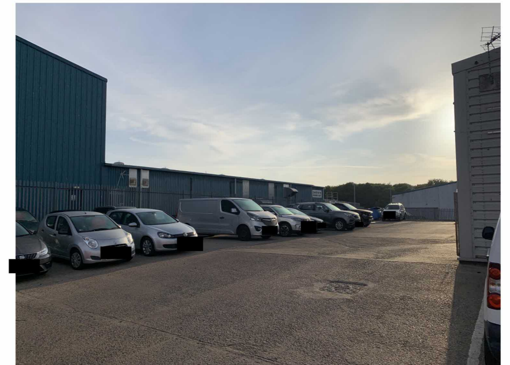
Photo 01 - Proposed location for new building
