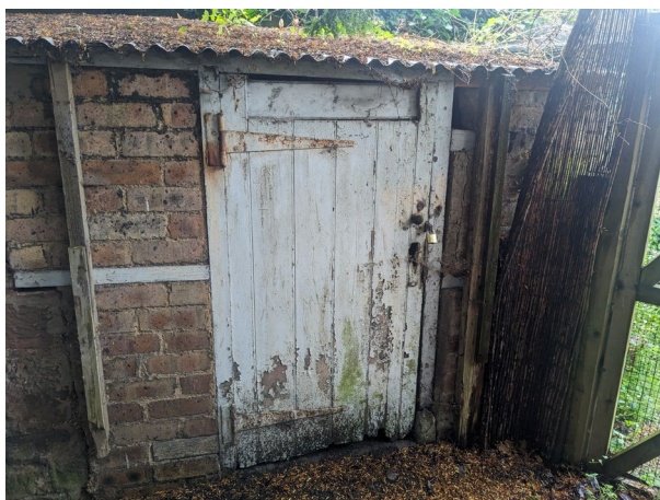
South Elevation – Last room at boundary.
