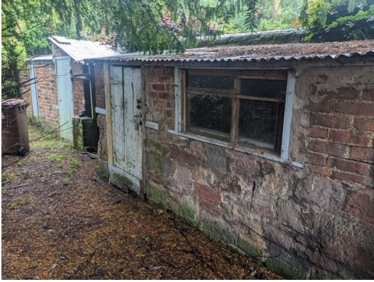
Figure 8 Single skin brick storage buildings
