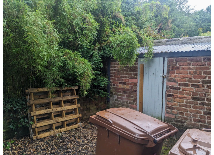
South elevation looking towards West room.
