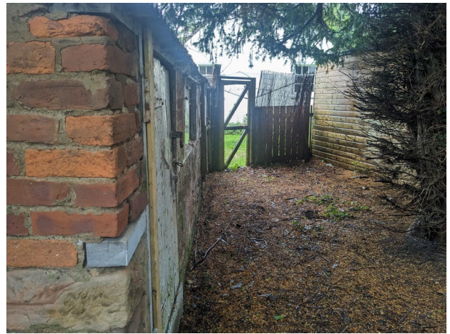
East towards boundary fence
